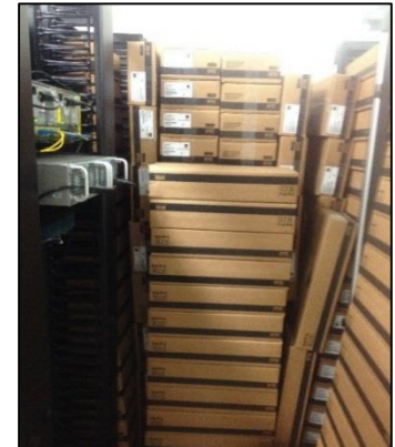
Boxes of storage in Data Center
