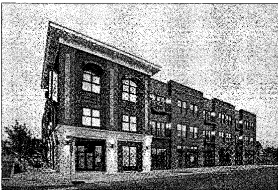
Example of a three story massing Hybrid Court with Shop Front configuration.
