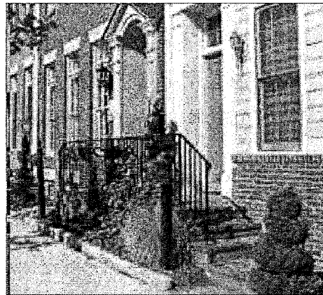
Example of Stoop serving two residential entries.
