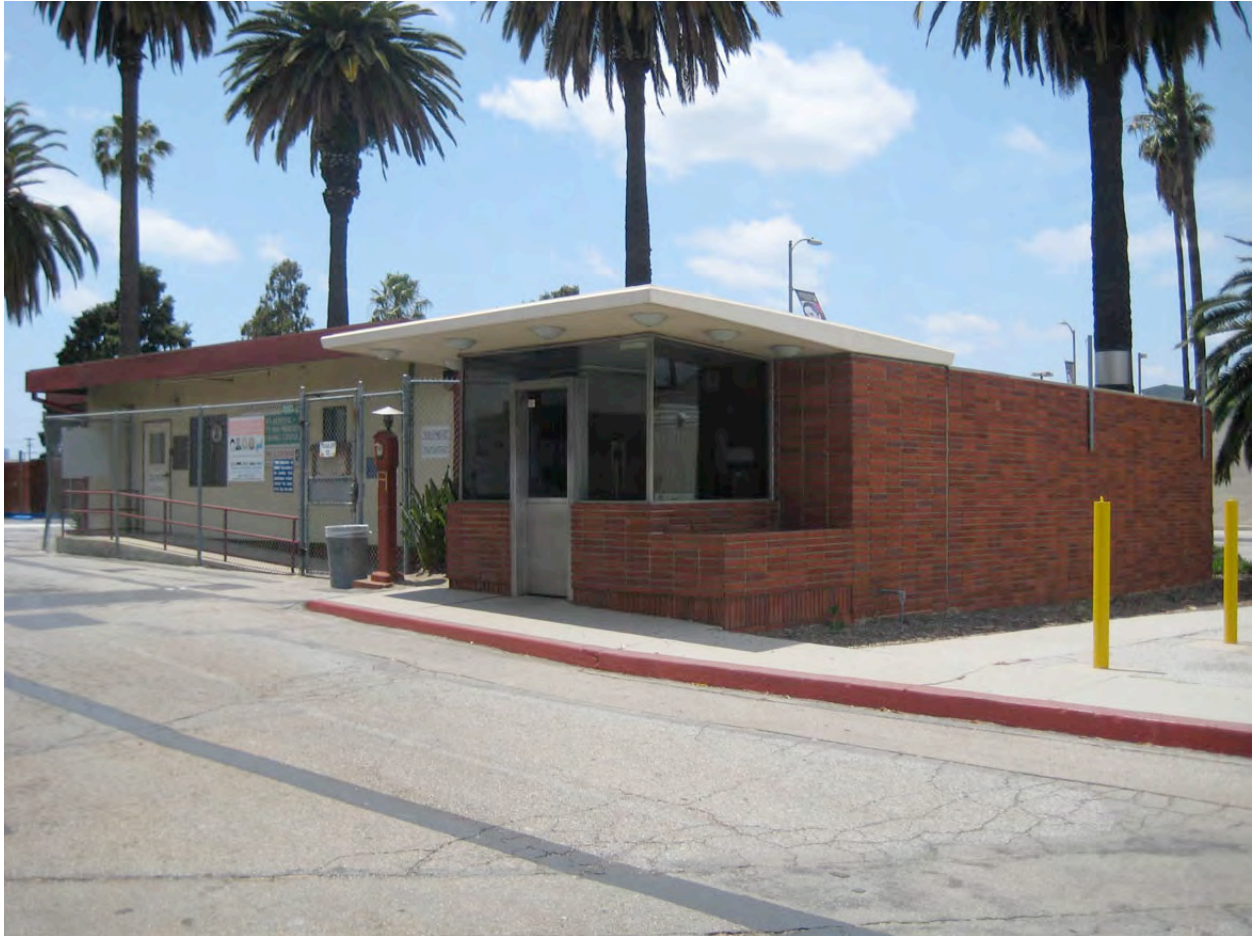
Photo 2: Gatehouse – Looking West/Southwest, Primary and Secondary Façade
