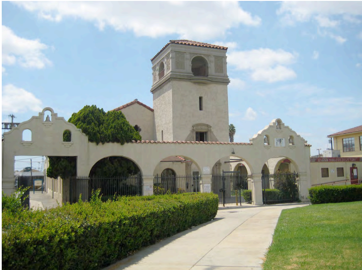
Photo 4: Building 30 – Looking West, Primary Elevation
