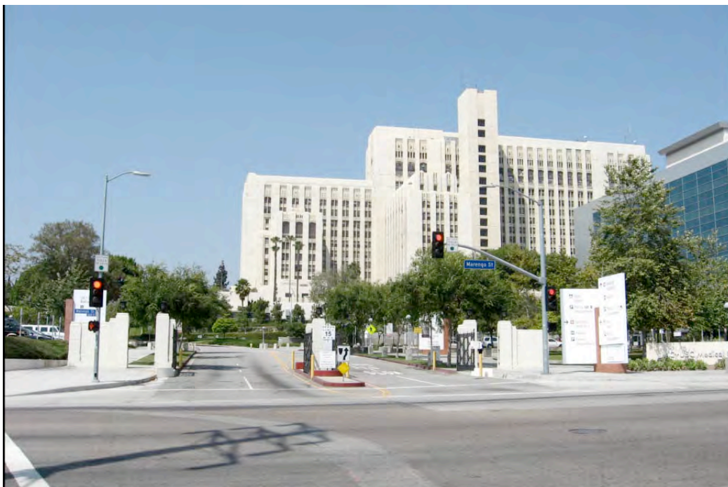
Photo 6: LAC+USC Medical Center Campus; View North from North State Street at Marengo Avenue Entrance
