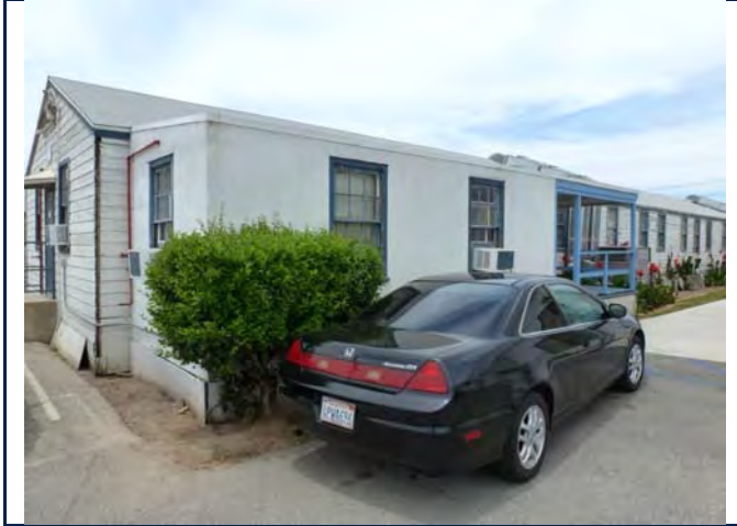
South and east elevations, view looking northwest. 6/11/13.
