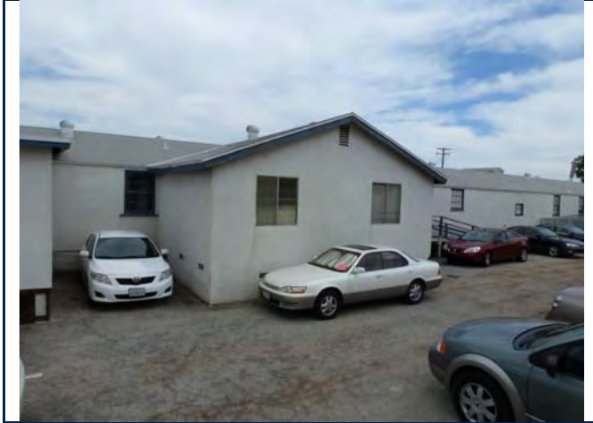
West elevation additions, view looking east. 6/11/13.
