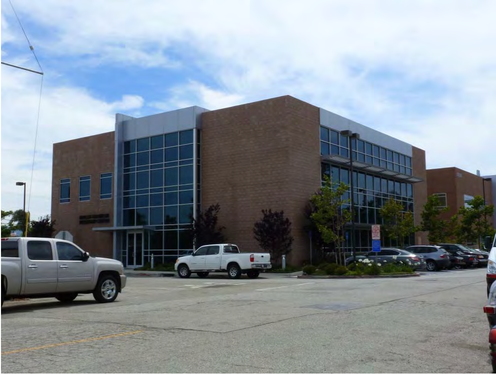
Figure 11: Hanley-Hardison Research Center, north and east elevations, view looking southwest. Source: GPA.
