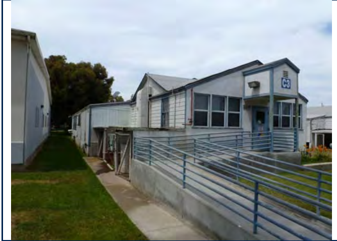
South and west elevations, view looking northeast. 6/11/13.
