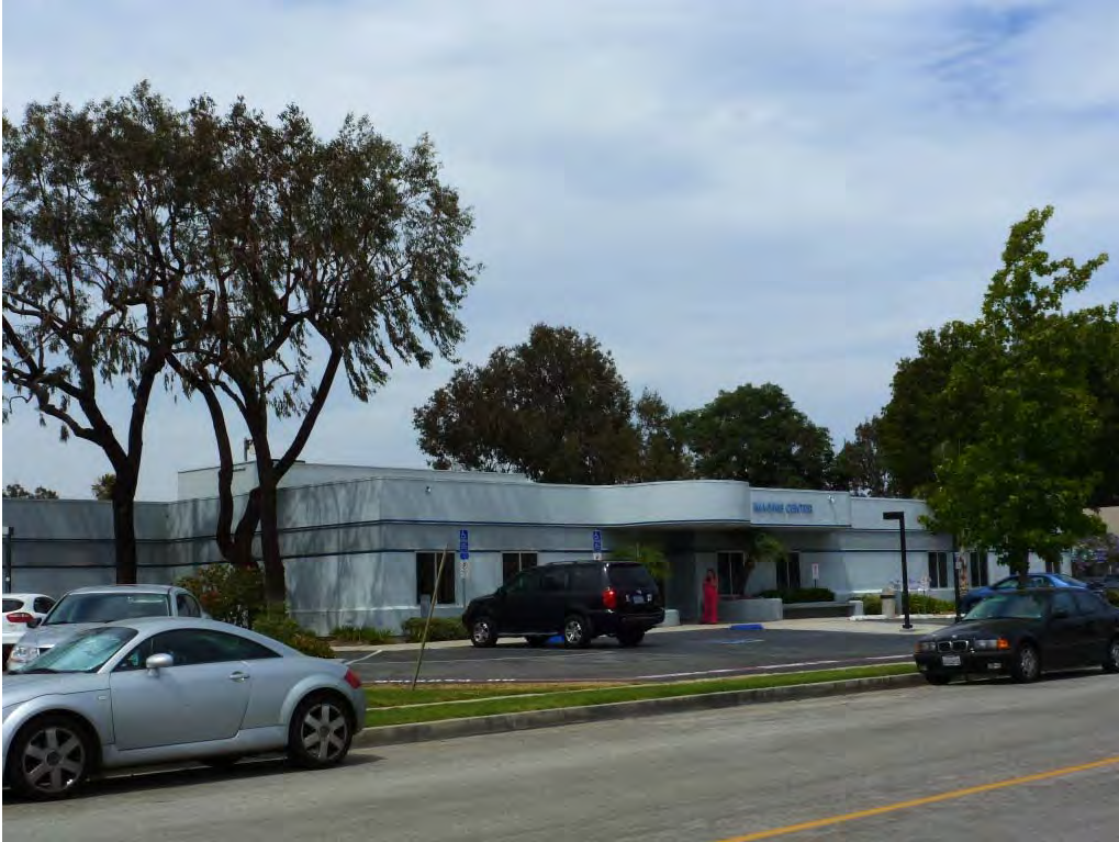
Figure 9: Imaging Center, view looking northeast. Source: GPA
