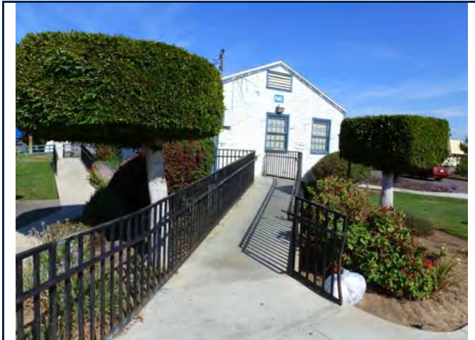
East elevation and ADA, view looking west. 6/11/13.
