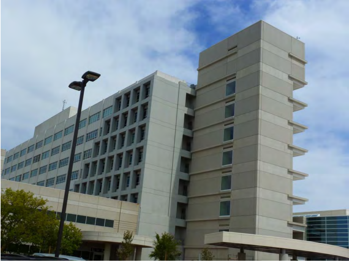
Figure 13: Hospital, north and west elevations, view looking southeast. Source: GPA
