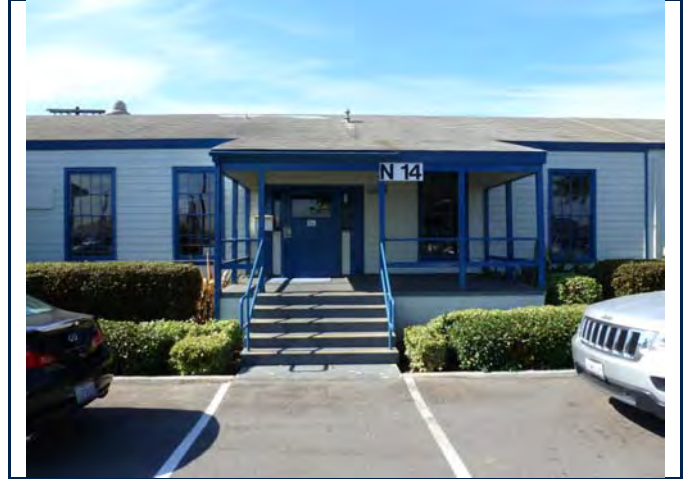
North elevation, west entrance. 6/11/13.
