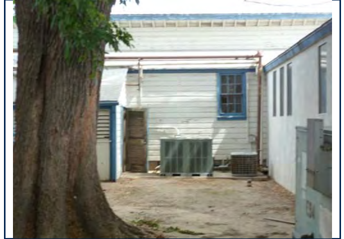
South elevation, view looking north. 6/11/13.
