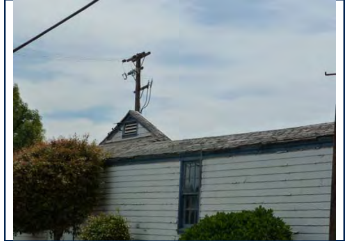
North elevation, gable remnant. 6/11/13.
