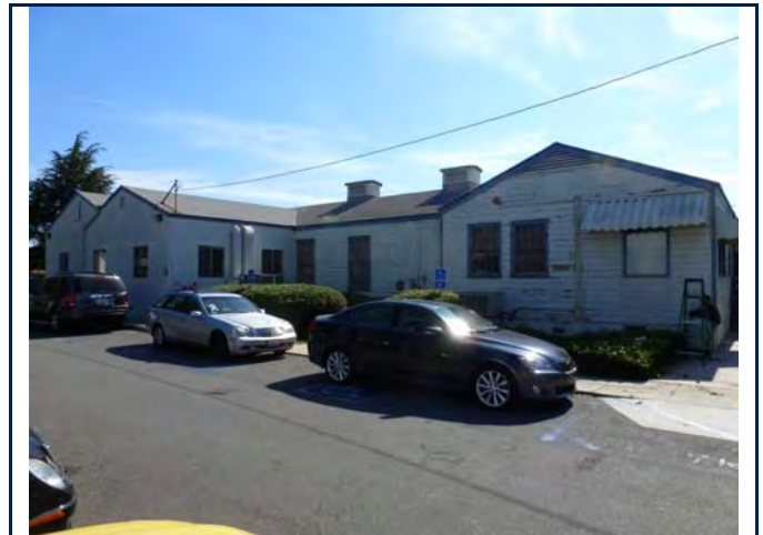
West elevation, view looking northeast. 6/11/13.
