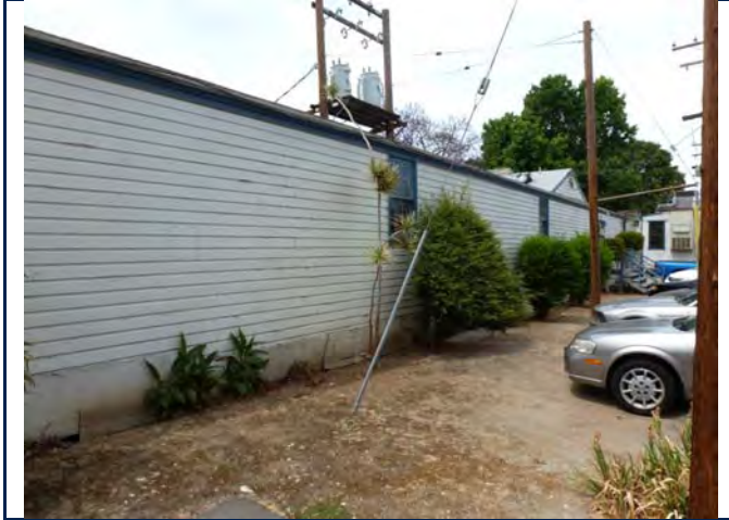
North elevation, view looking southwest. 6/11/13.
