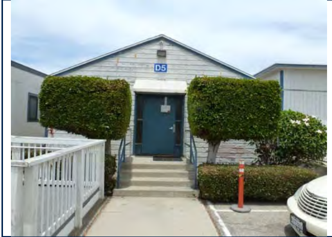
South elevation, view looking north. 6/11/13.
