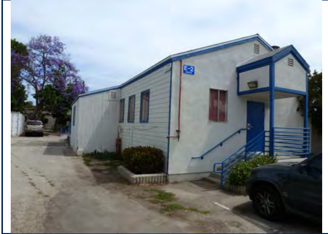
South and west elevations, view looking northeast. 6/11/13.
