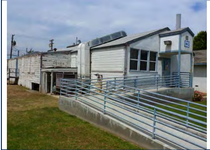
South and west elevations, view looking northeast. 6/11/13.
