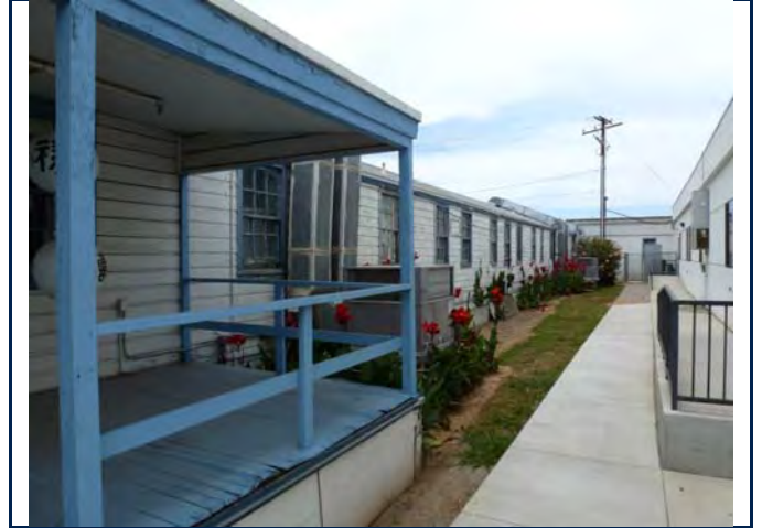
East elevation, view looking northwest. 6/11/13.
