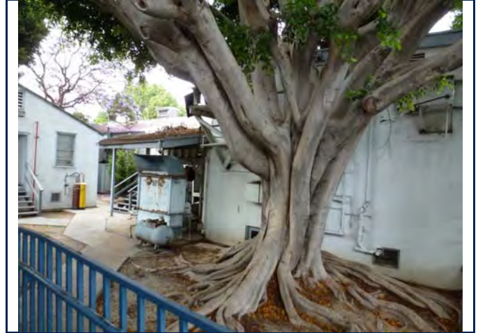
West elevation, south end, view looking northeast. 6/11/13.
