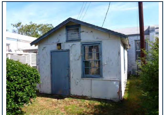
South elevation, free-standing shed. 6/11/13.
