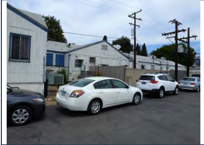
East elevation, view looking north. 6/11/13.
