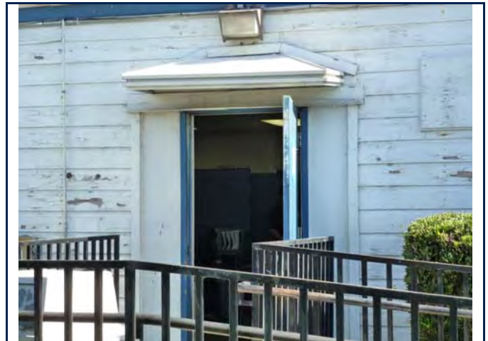
South elevation, entrance. 6/11/13.
