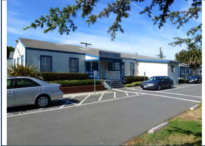
North elevation, east end, view looking southwest. 6/11/13.
