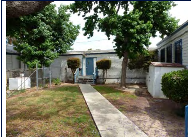
South elevation, view looking north. 6/11/13.
