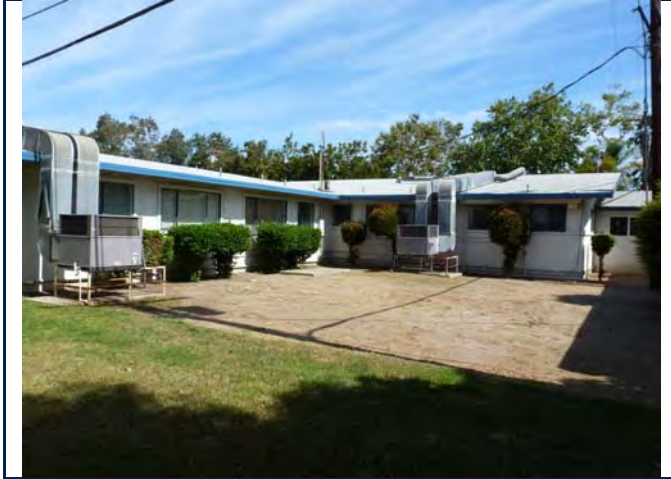
South and east elevations, view looking northwest. 6/11/13.
