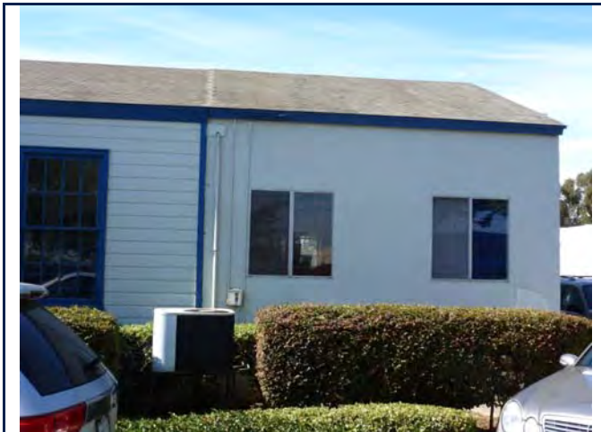
West elevation, addition detail. 6/11/13.
