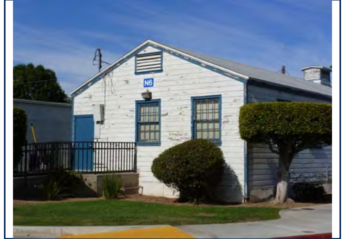
East elevation, view looking southwest. 6/11/13.
