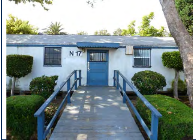
North elevation, entrance. 6/11/13.
