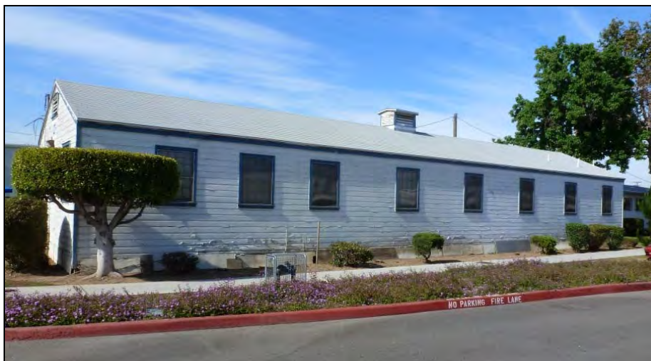
Figure 3: Building N6, north elevation, view looking southwest. Source: GPA.
