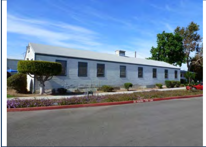
North elevation, view looking southwest. 6/11/13.
