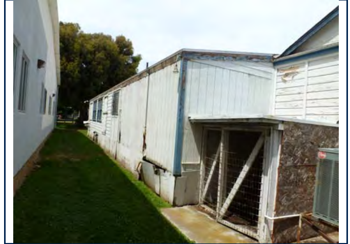
West elevation, view looking northeast. 6/11/13.
