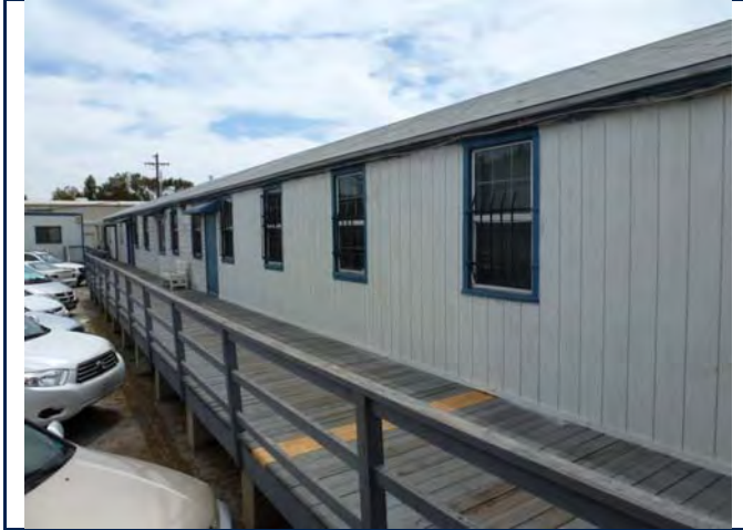
East elevation, view looking southwest. 6/11/13.
