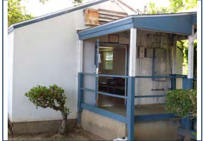
West elevation, view looking southeast. 6/11/13.
