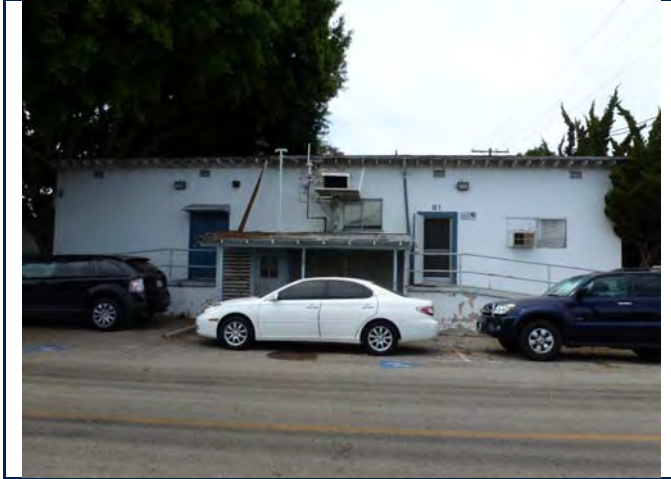
South elevation, view looking north. 6/11/13.
