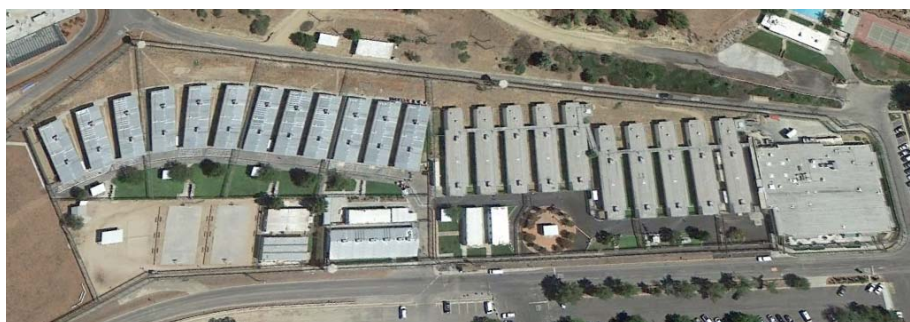
Figure 1.8: Pitchess Detention Center (South) Site
