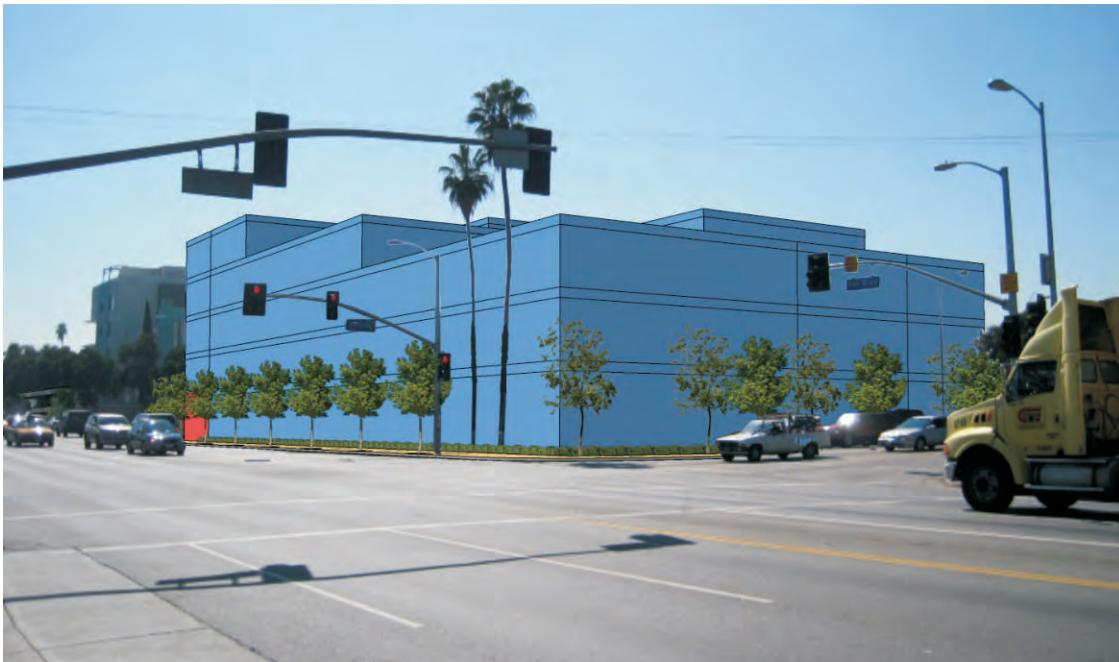
Proposed Conditions: View of the northeast corner of the project site from Van Nuys Boulevard/Saticoy Street intersection.
