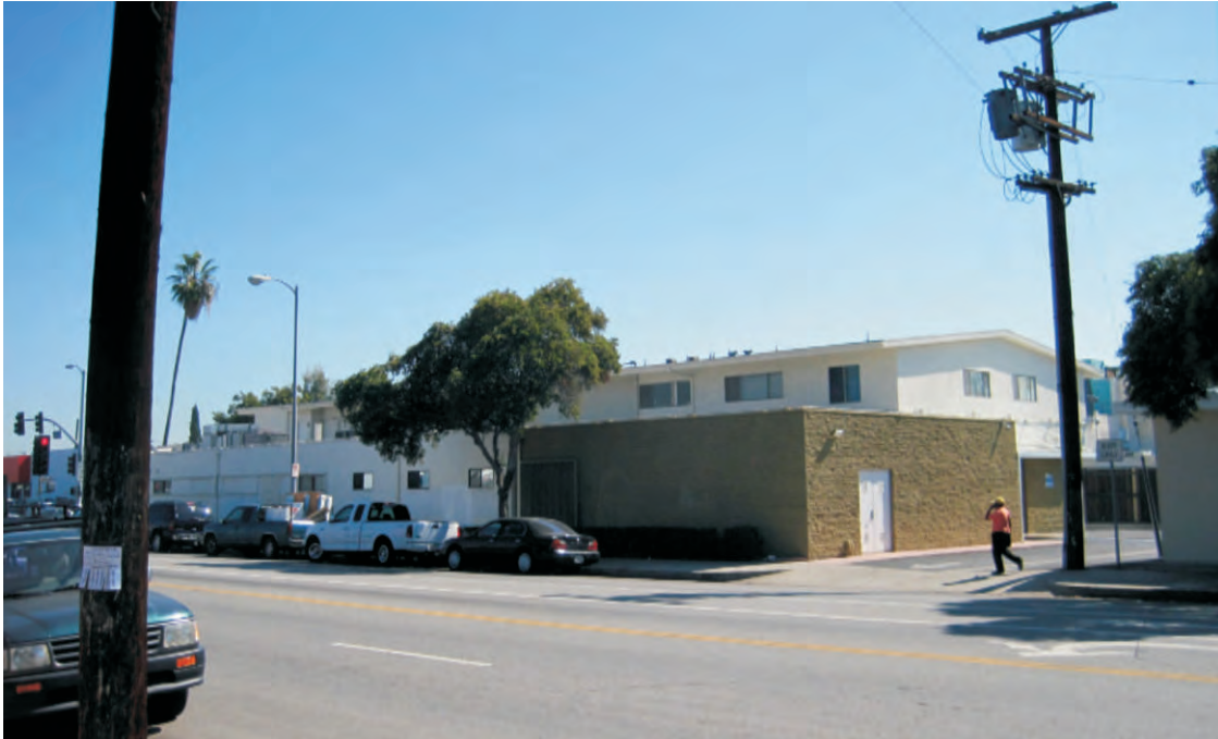
Existing Conditions: View of the northern project boundary from Saticoy Street.
