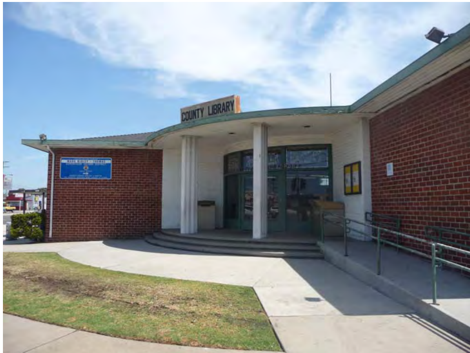
Library, Primary (south) elevation, view north (PCR 2011)
