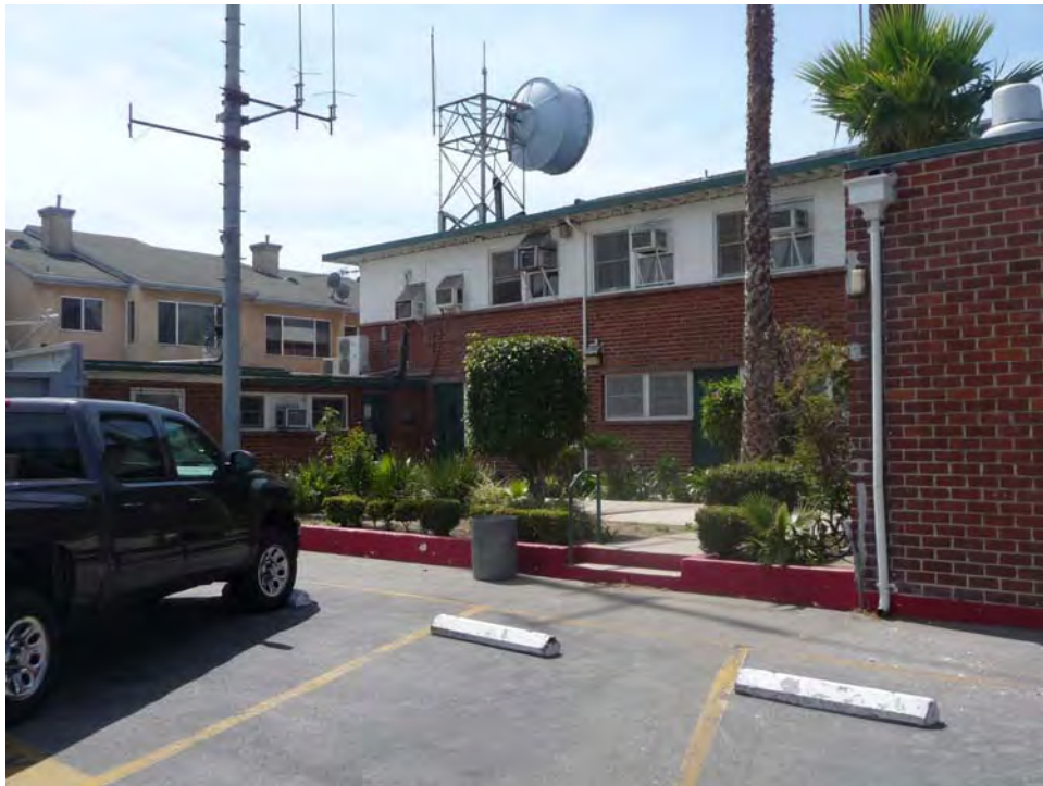
North elevation, view south (PCR 2011)
