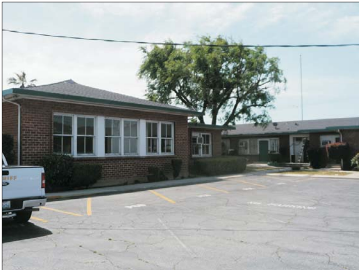
Photograph 7: County Office Building, Rear (Northern) Elevation and Courtyard.
