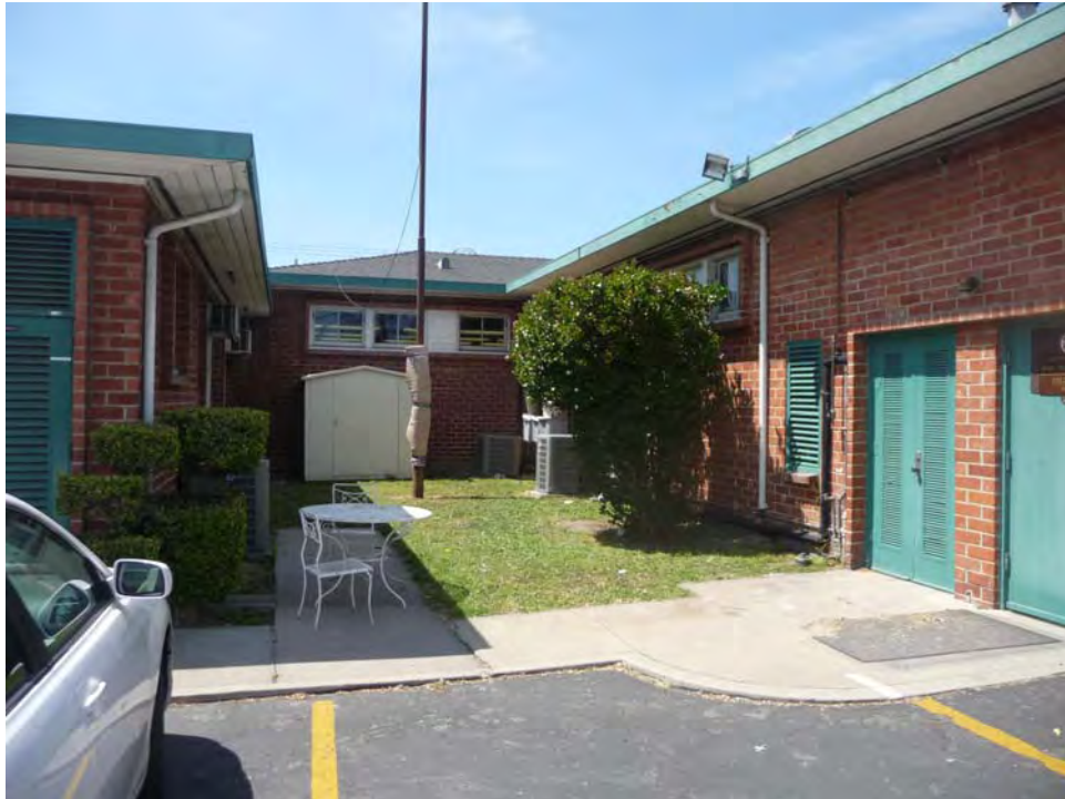
North elevation, view south (PCR 2011)
