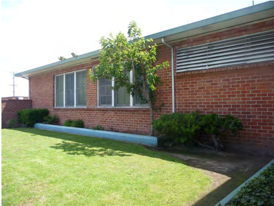
Library, west elevation, view east (PCR 2011)
