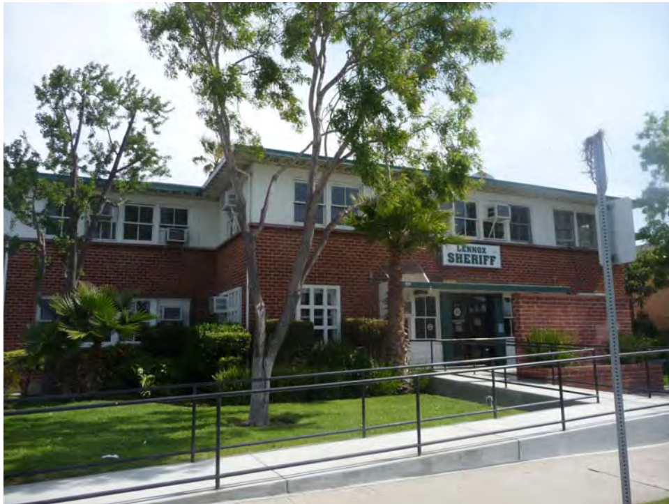
Sheriff's station, Primary (south) elevation, view to north (PCR 2011)
