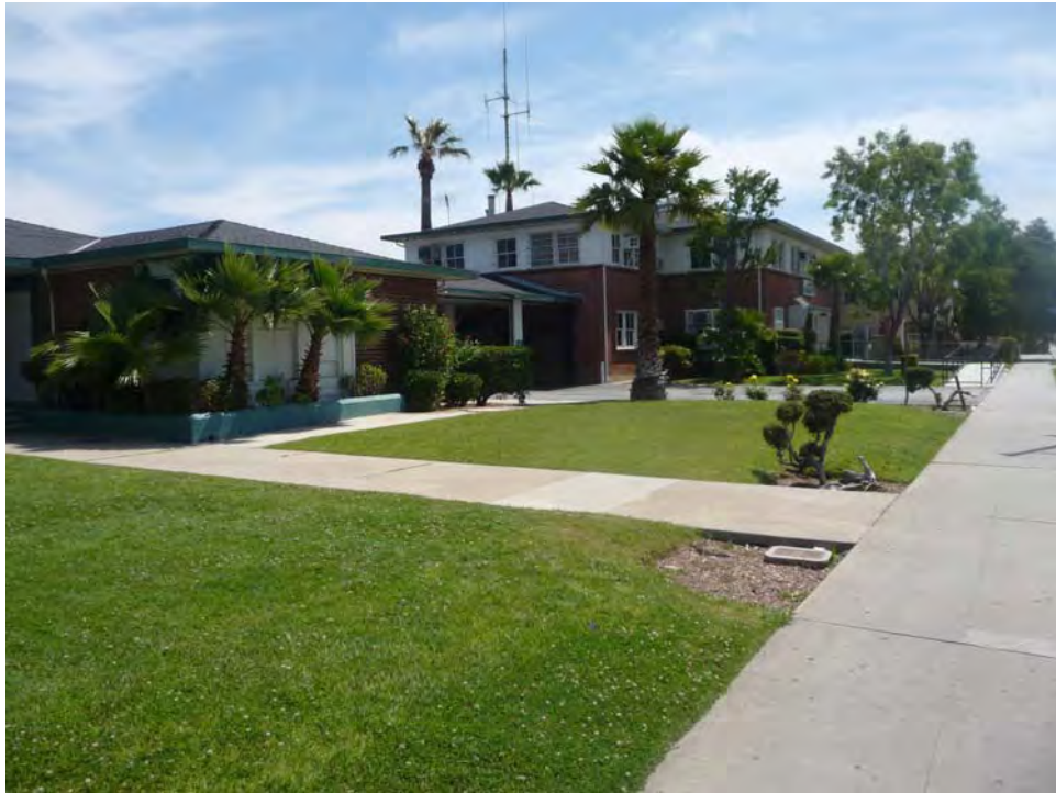
Primary (south) elevation, view north (PCR 2011)
