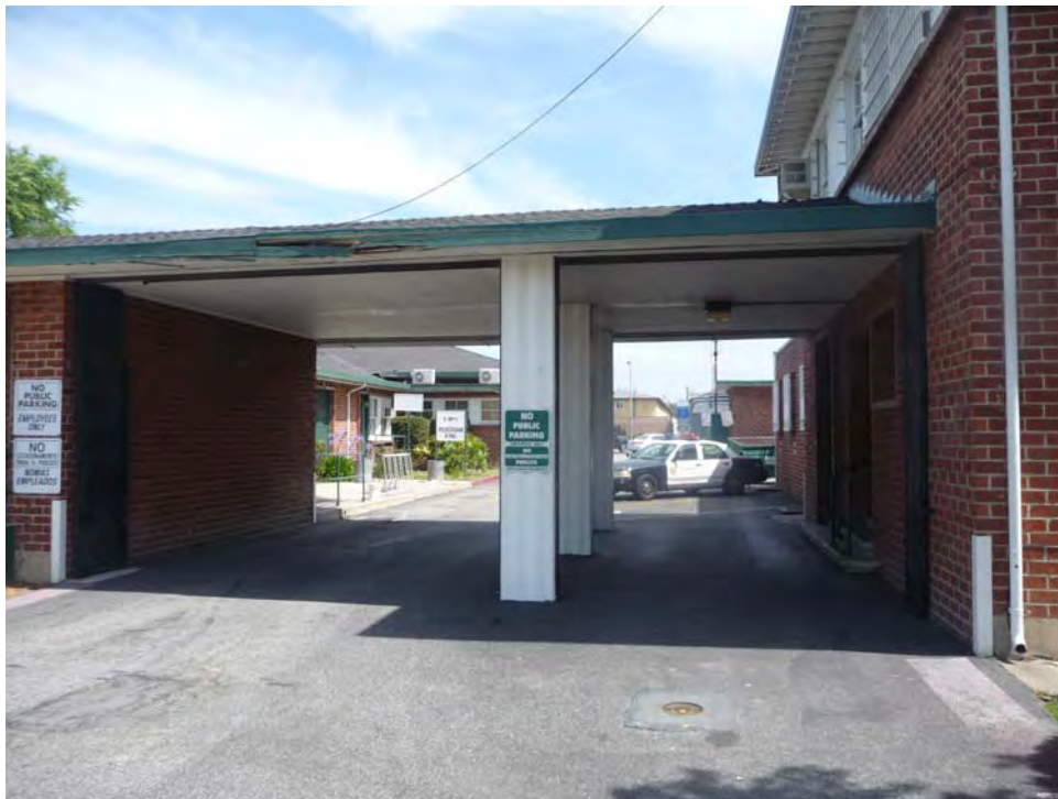
Carport, South elevation, view to north (PCR 2011)
