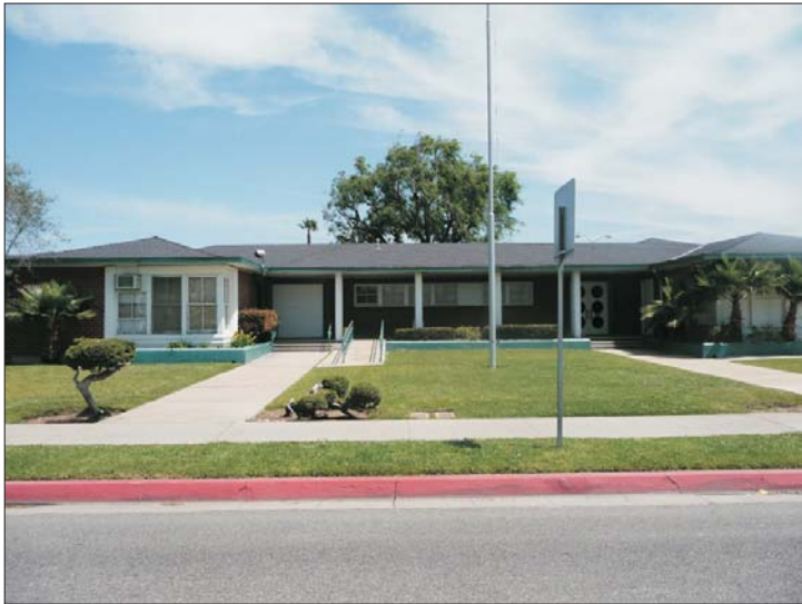
Photograph 3: County Office Building - View from Lennox Boulevard.
