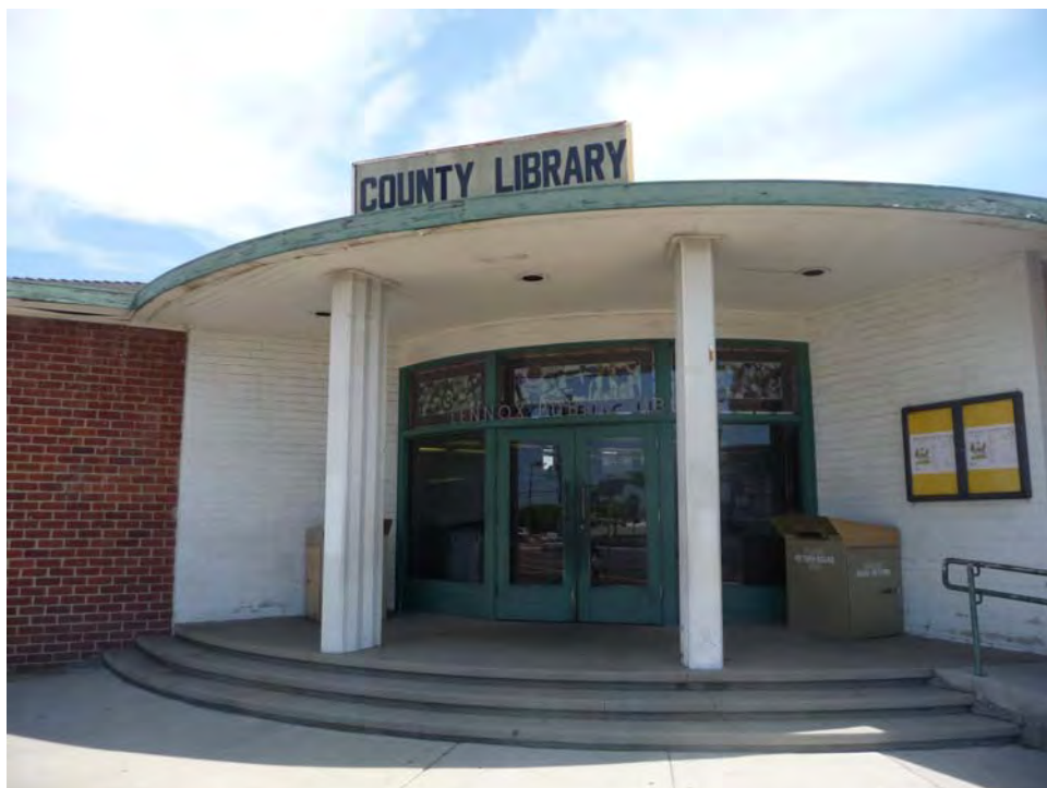
Library, Primary (south) elevation, view north (PCR 2011)
