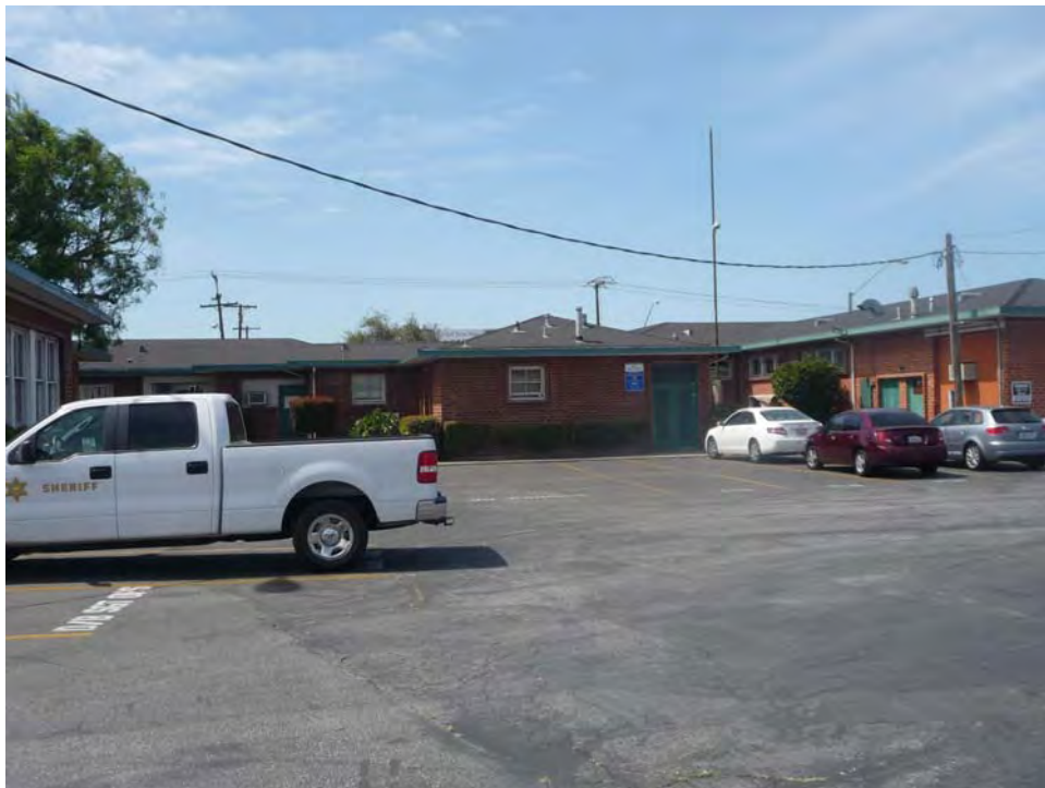
North elevation, view south (PCR 2011)
