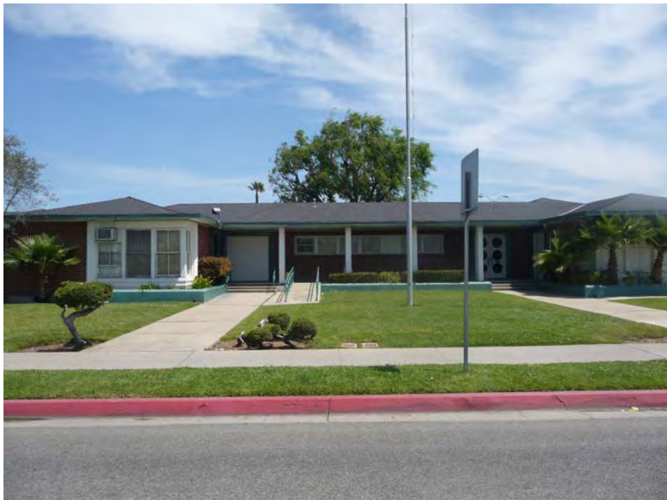
Primary (south) elevation, view north (PCR 2011)
