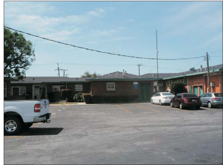
Photograph 6: Library, Rear (Northern) Elevation and Parking Lot.
