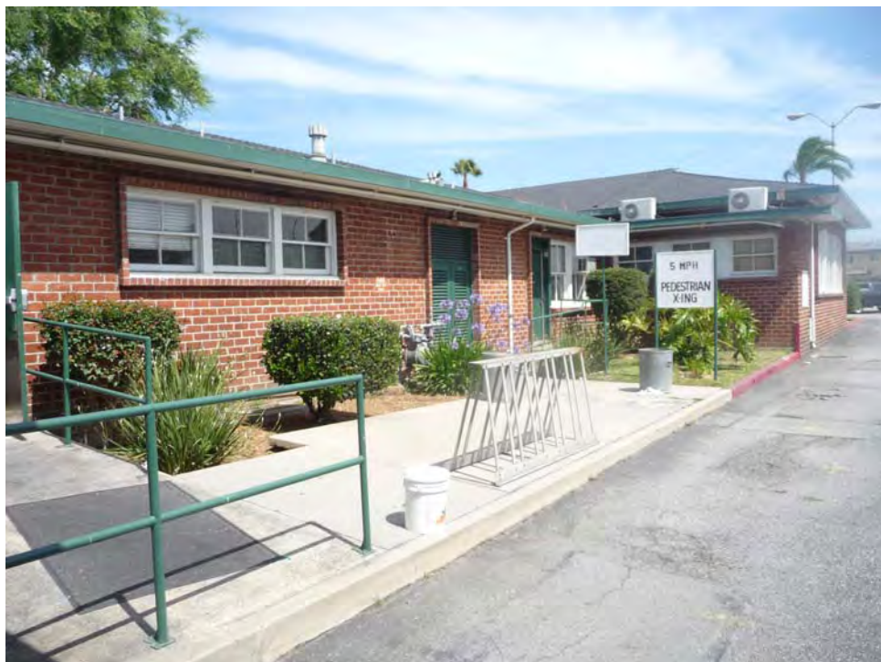
Department of building and safety, east elevation, view northwest (PCR 2011)
