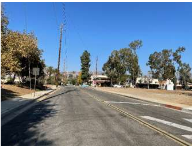
CATARACT AVE., LOOKING NORTH
