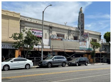
Figure 1. Primary Façade (CDF 3: cornice coping; CDF 5: glazed brick, pilasters, parapet roofline, glazed brick stringcourse) SOURCE: Sapphos Environmental, Inc., 2021
