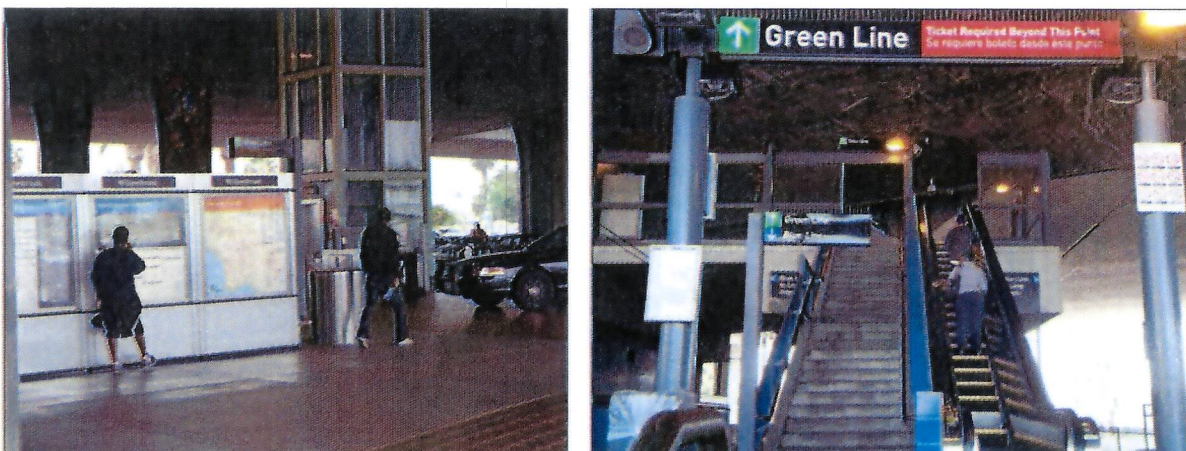
The Willowbrook/Rosa Parks Station environment is inhospitable and unattractive.
