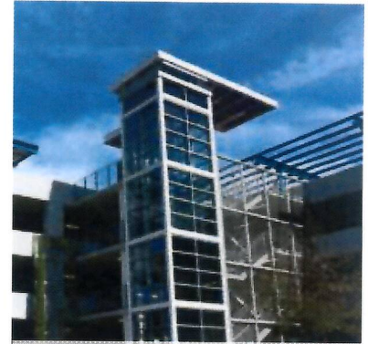
Example photo illustrating a parking structure with architectural and screening features.
