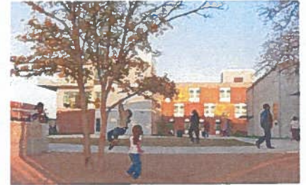
A community playground at Haven for Hope, TX campus. Source: Overland Partners, Accessed from https://www.overlandpartners.com/projects/haven-for-hope-homeless-transformational-center/
