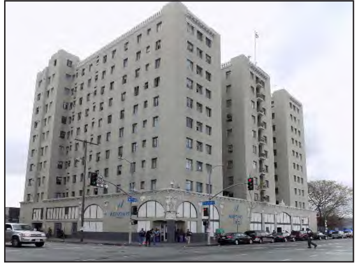
View 6: View looking northeast on the intersection of San Pedro Street and 6th Street at the Weingart Tower across from Site 2.
