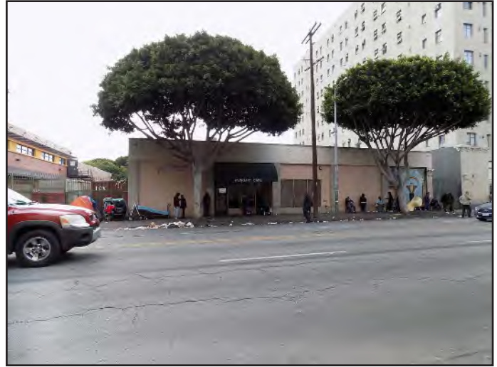
View 2: View looking southeast along San Pedro Street at Site 1.
