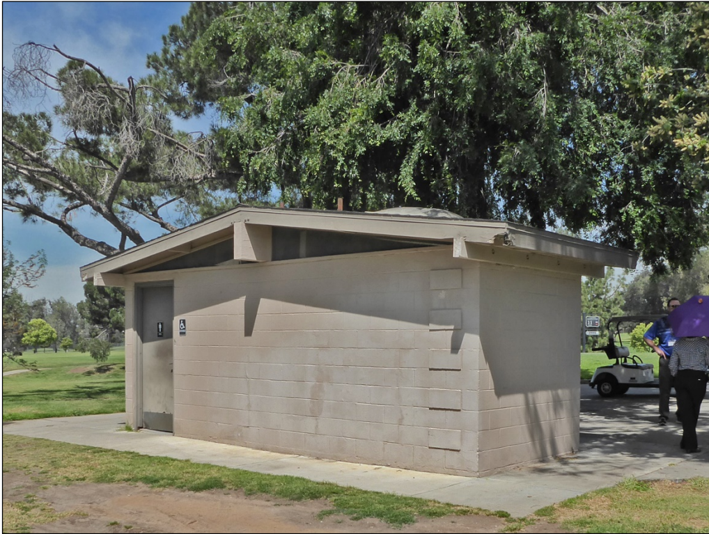
Figure 20. Comfort Station No. 2, entrance to men's restroom.
