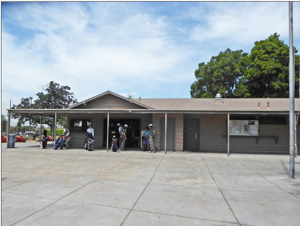
Figure 15. Pro Shop, view toward the primary entrance.
