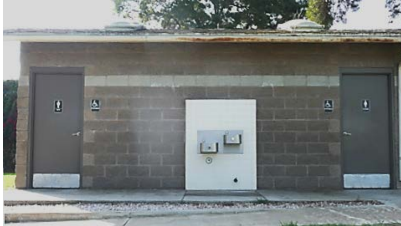
Figure 9. View of Comfort Station No. 1, Chester Washington Golf Course SOURCE: Sapphos Environmental, Inc., 2016
