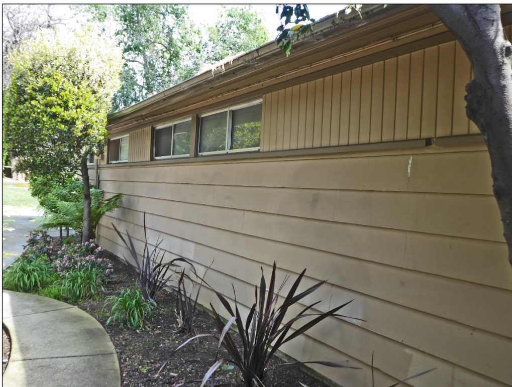
Figure 17. Exterior siding of Pro Shop.
