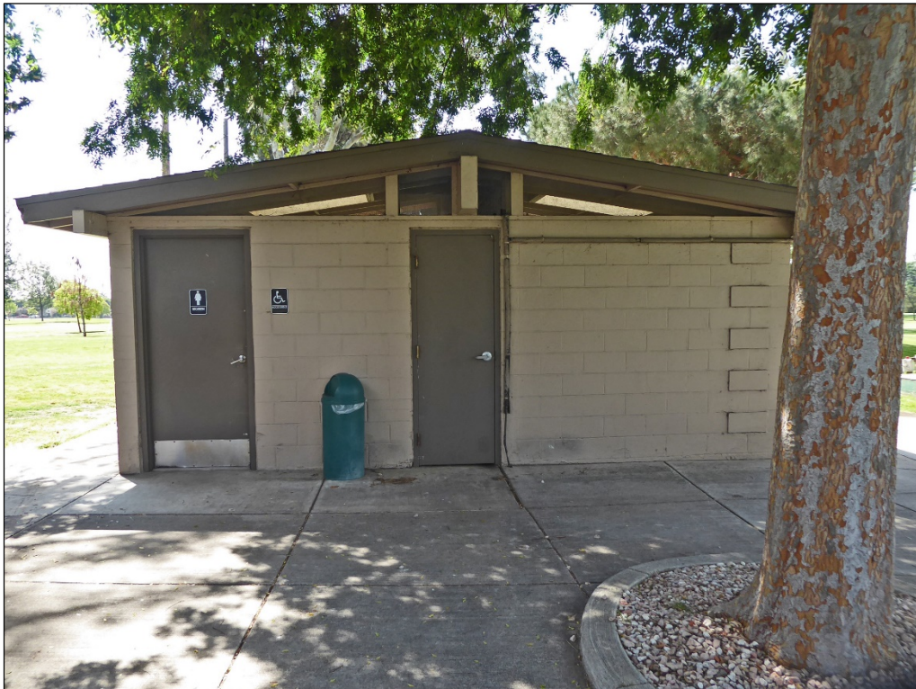
Figure 19. Comfort Station No. 2, entrance to women's restroom.
