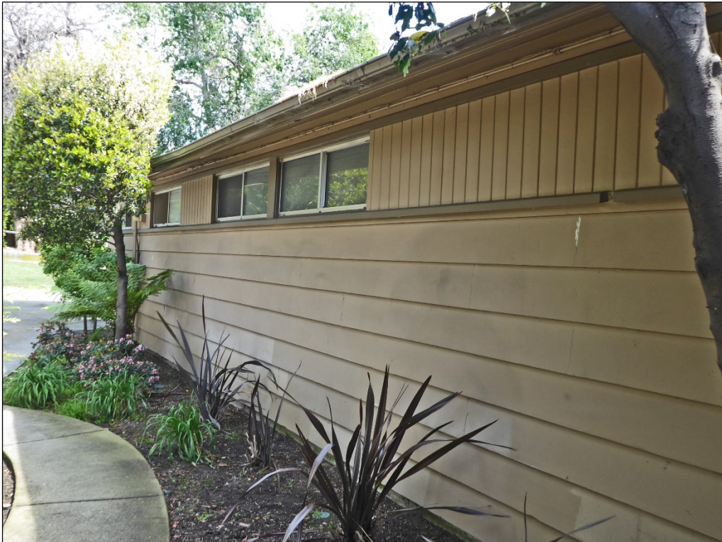
Figure 17. Exterior siding of Pro Shop.
