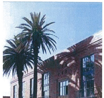
Example photo illustrating a building aligned with the right-of-way.
