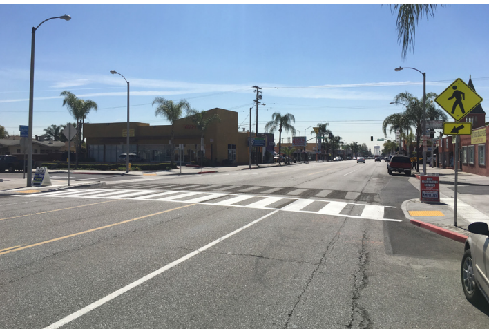
A ladder crosswalk with accessible curb ramps and curb extensions in Walnut Park
