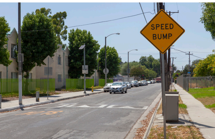
A typical speed hump, supplemented with speed hump signage and pavement markings
