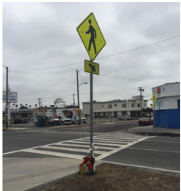
Unsignalized crosswalk at the intersection of Vermont Avenue and 94th Street, where the project team observed motorists not yielding to pedestrians
