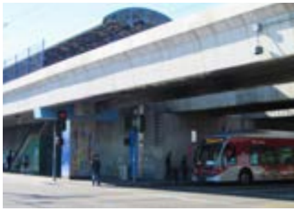
Firestone Station elevated platform.
