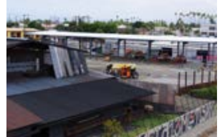
Industrial facilities in the process of being upgraded.
