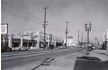
Florence Avenue retail corridor near Holmes Avenue, 1952.
