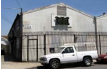
Industrial use in Florence-Firestone with well-maintained façade and fencing.
