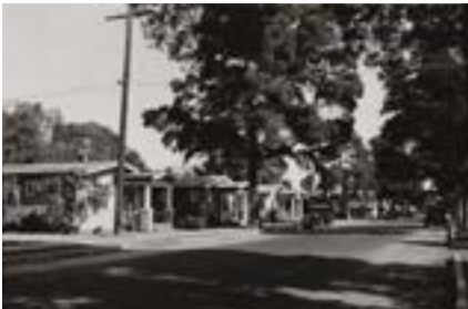
Residence on 70th St., between Compton and Makee, 1932-1933. Courtesy, California Historical Society
