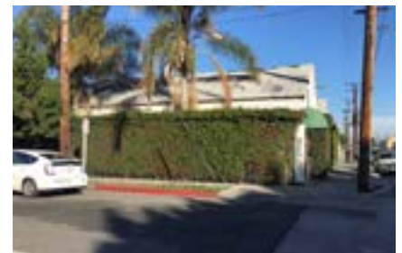
Industrial use on Wilmington Avenue with landscaping and fencing.
