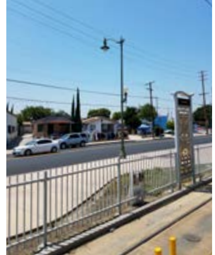
Example of dual purpose street- and pedestrian-scale lighting on one pole. Courtesy, Daryl Koonce
