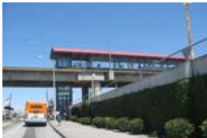
Industrial use on Slauson Avenue with landscaping and walls for buffering and screening.
