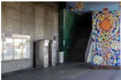
Firestone Metro Station.
