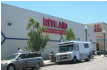
The Rite-Aid on Florence Avenue does not provide an entrance from Florence Avenue and is not oriented to the street.
