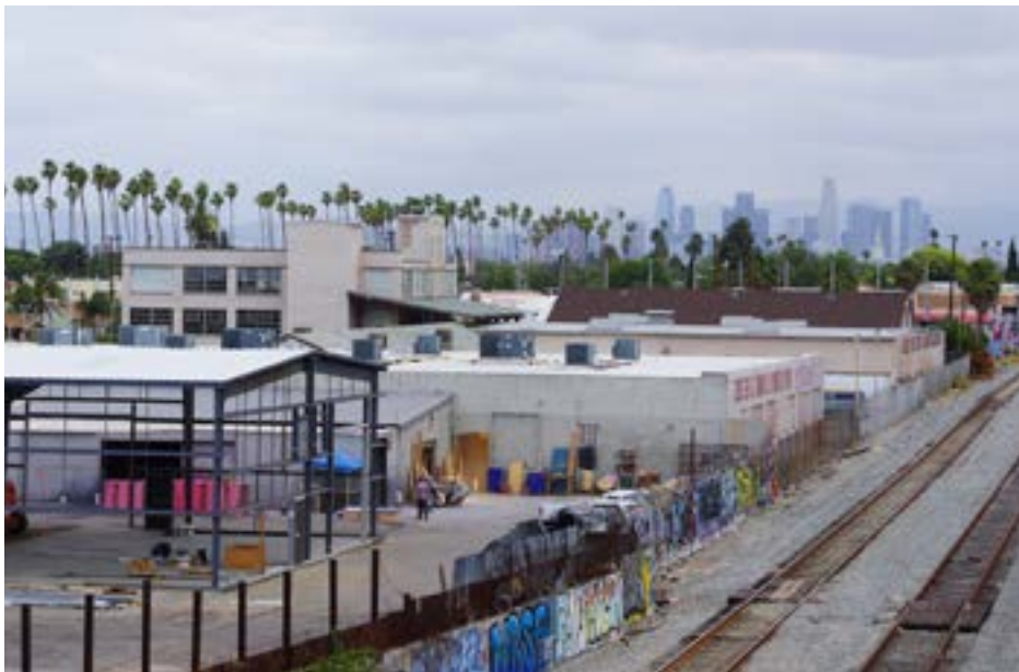
Metro Blue Line and railroad rights-of-way with graffiti on walls.
