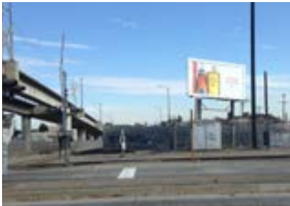
Poor pedestrian amenities at Slauson Station.
