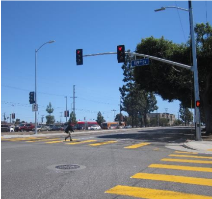
Existing pedestrian crossing.
