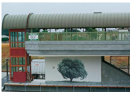
Existing view of transit station boarding area.
