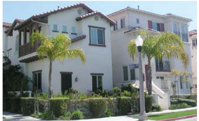
Example of multi-family residential development.
