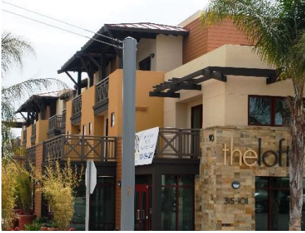
Illustrative photo of building modulation and articulation.
