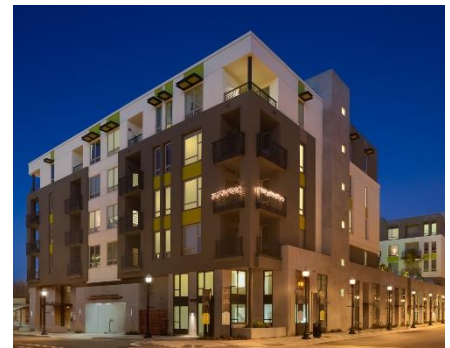
Illustrative photo of architecturally compatible lighting.
