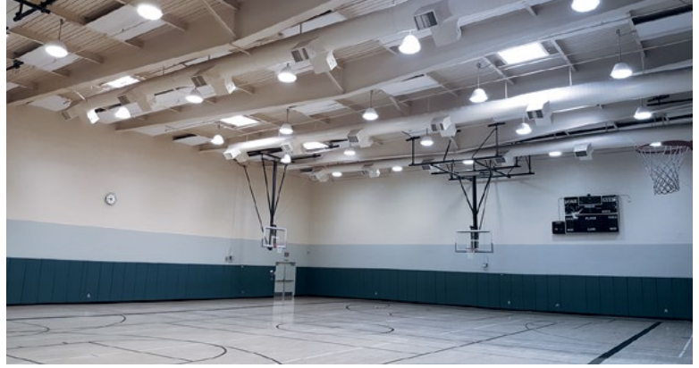
Interior lighting upgrades at a municipal basketball court in Palmdale.
