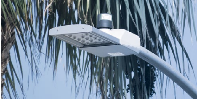
LED street light upgrade in The City of Orange
