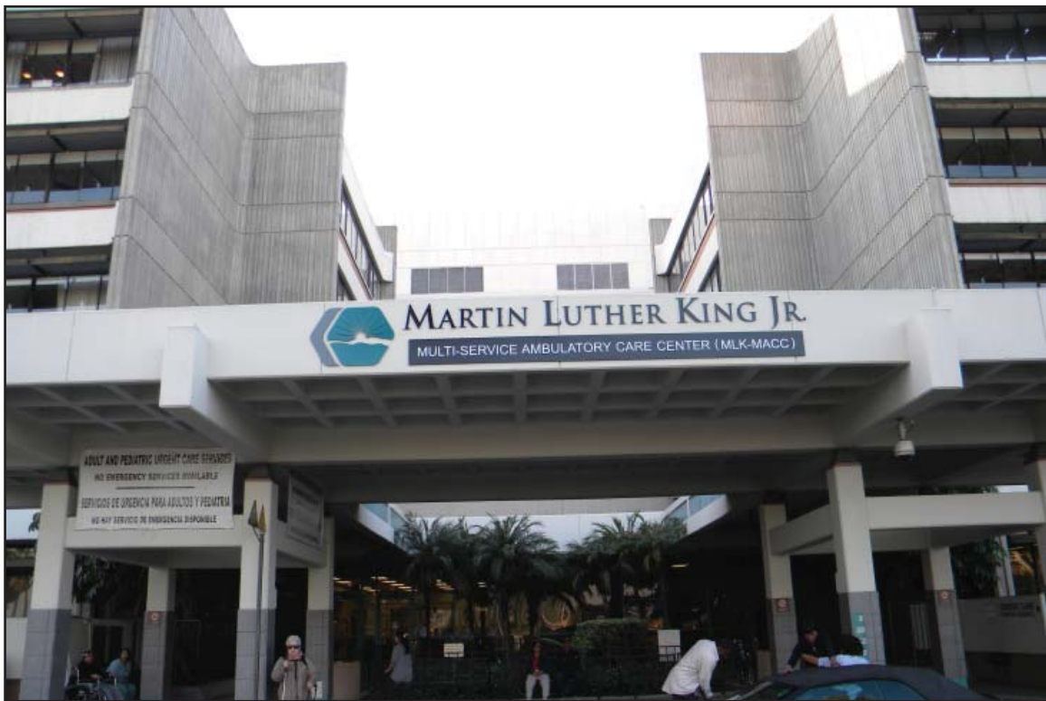
KVP 1: View of main entrance of the MACC five-story building. View from the east looking west at existing structure
