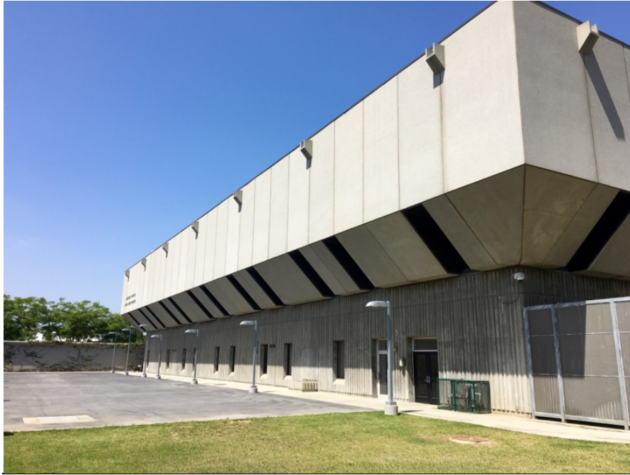
Figure 7 View of Hawkins Building looking Northeast
