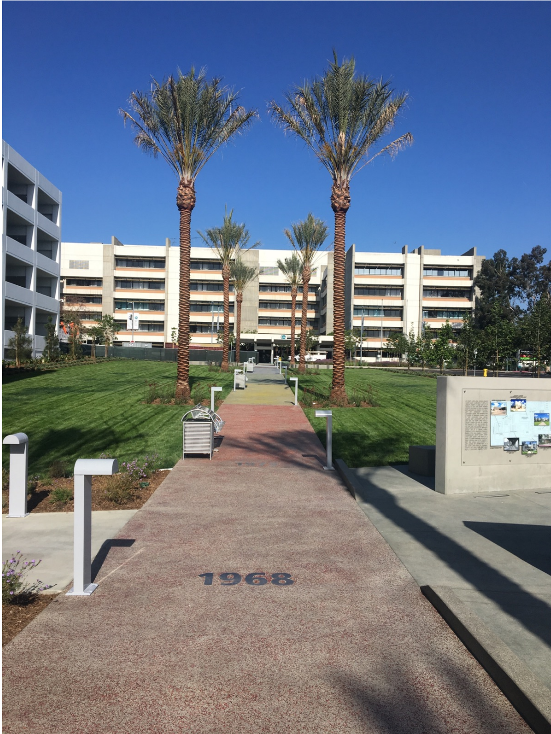
Figure 4 View West of Original MACC (Future BHC) and Reconfigured Green Area
