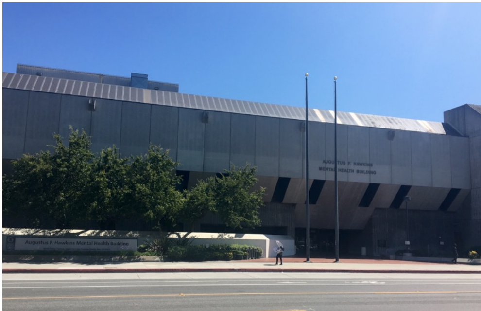
Figure 6 View of Hawkins Building looking South from 120th Street
