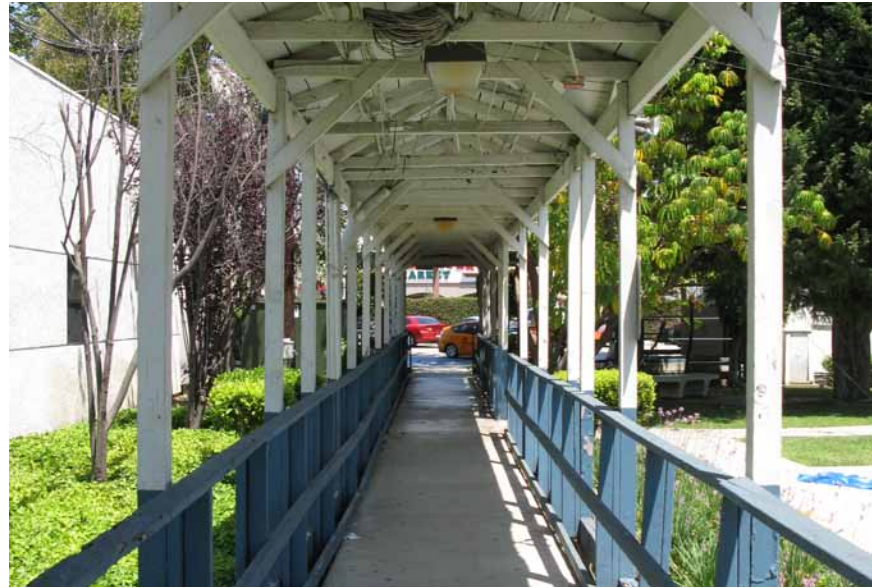
Canopy connecting modular buildings
