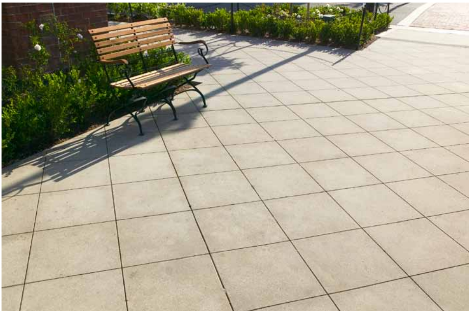
Integral color concrete paving with sawcut joints
