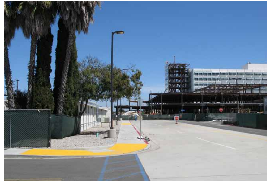
New Emergency Department construction
