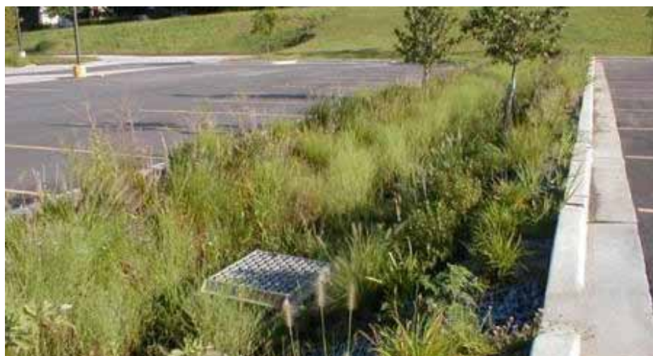
Central curb cut in parking island collects stormwater runoff.
