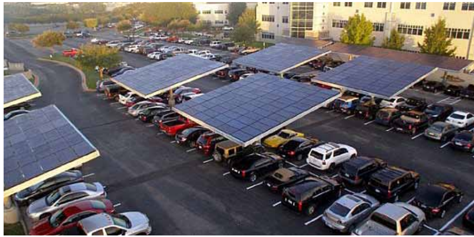
Photovoltaic panels shading parking areas
