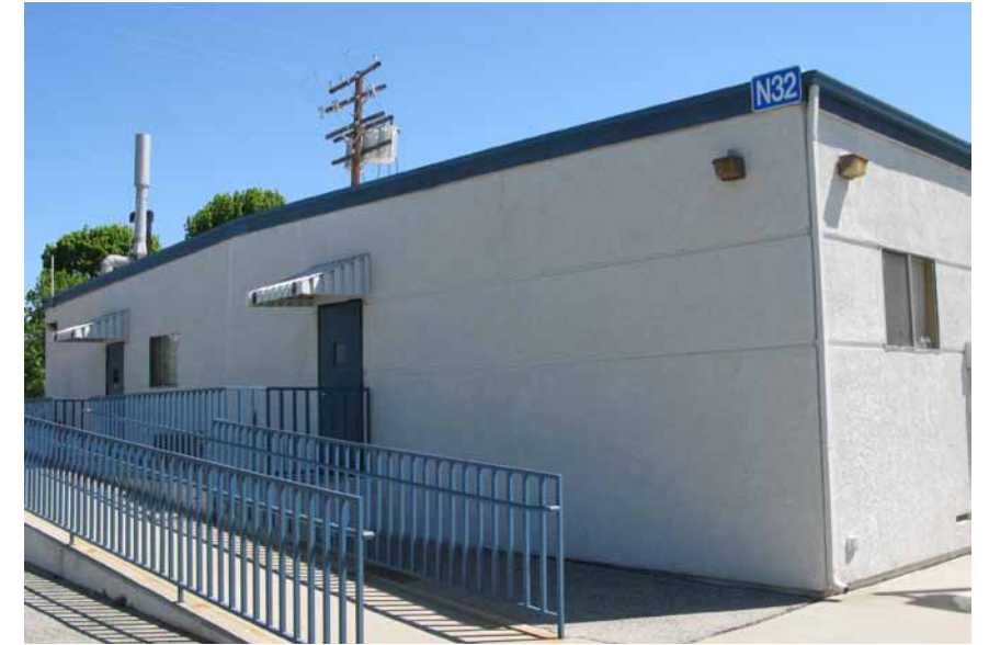
Building N32 - Typical modular building
