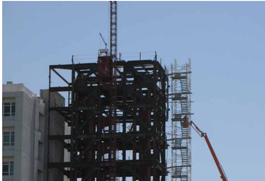
New elevator connection to Existing Hospital Tower
