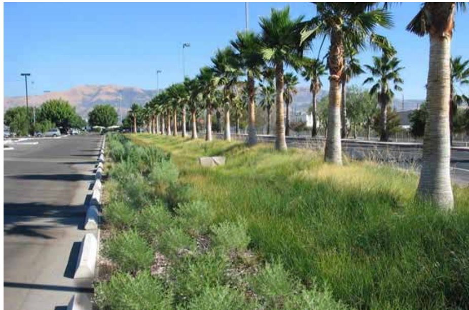
Vegetated swale in a zero curb parking area
