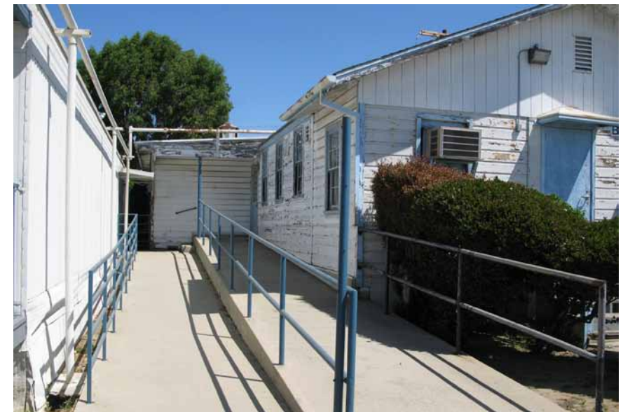
Accessible ramps interfacing with WWII modular buildings
