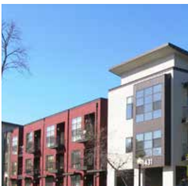
Example photo illustrating the use of colors and materials that are consistent with an overall architectural theme.
