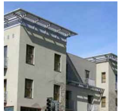
Example photo illustrating a roof style that complements the architecture and screens mechanical equipment.
