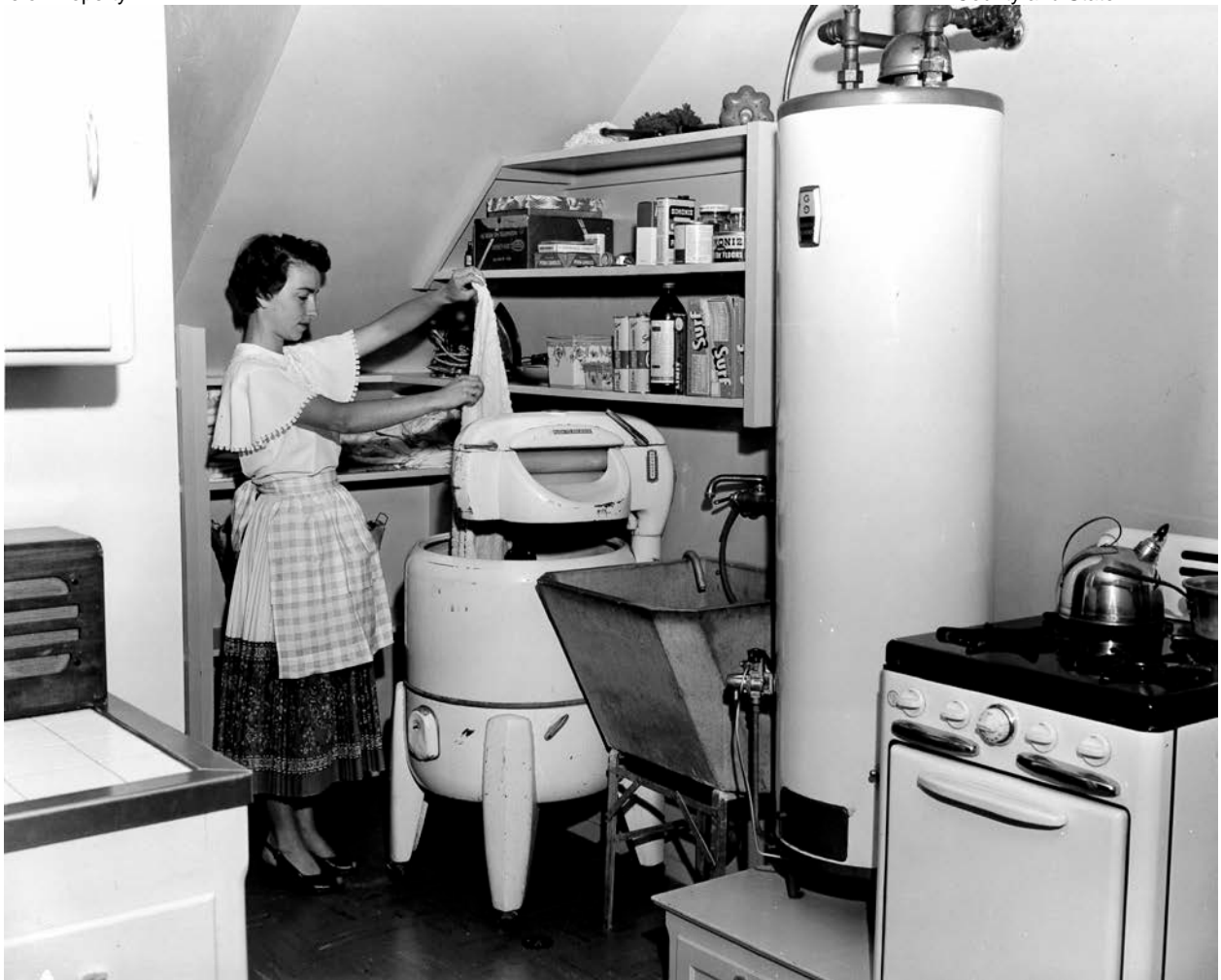
Figure 4: “Interior View, Kitchen and Service Room. Mrs. Patricia Lopez, 11844 ½ Allin Street.” (Building No. 7, Type E). Undated. Courtesy of HACLA.
