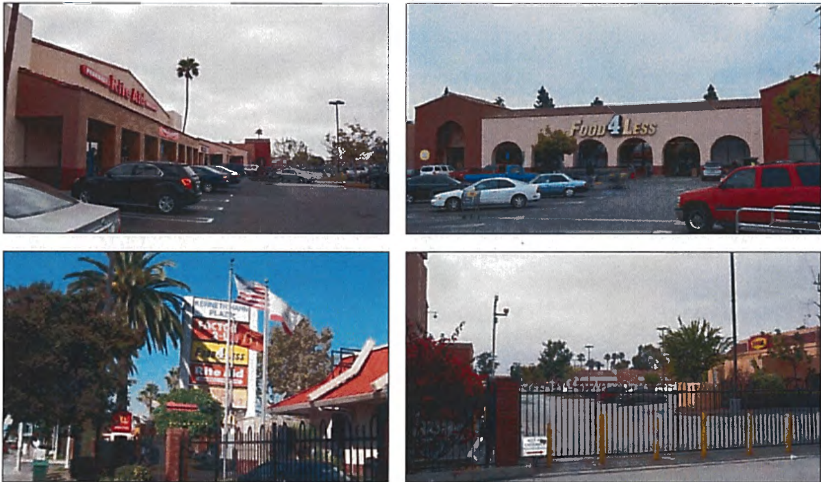
Kenneth Hahn Plaza currently has neighborhood serving retail as anchors. It is also isolated from its surroundings by fencing.
