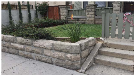
Figure 6. Photo 0010 Cast Stone Wall Detail
