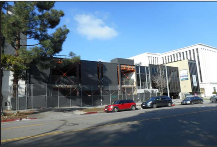
View 10: New Office Building Under Construction North of Site 1 Parking Structure on Shatto Place.
