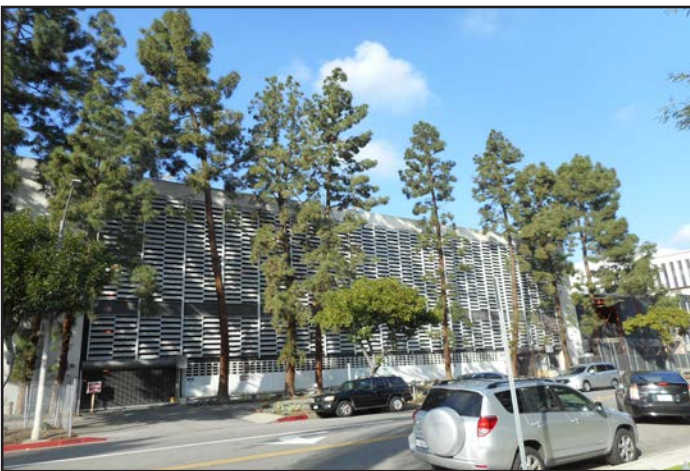
View 6: Parking Structure Serving County Office Buildings.
