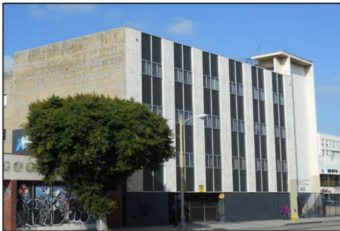
View 3: DPR Building Viewed from Southeast.
