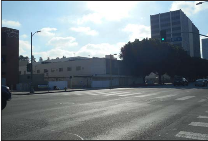
View 1: County DPR Building.
