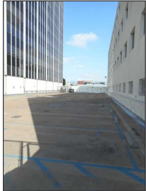
View 5: Surface Parking Lot between DMH Building and CSS Building.
