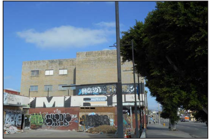
View 2: DPR Building Viewed from South.
