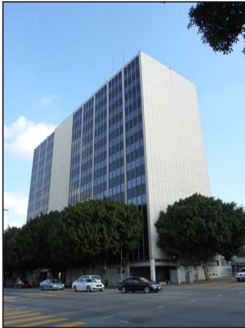
View 1: DMH Building.
