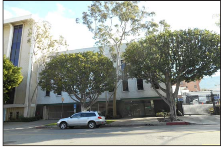
View 11: Office Building Located East of Site 1 Parking Structure Across Shatto Place.
