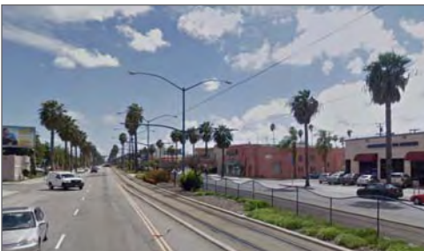
The Blue Line provides excellent regional transit access, but it also creates east–west barriers and adds over 20 feet to an already wide roadway with its exclusive travel lanes.
