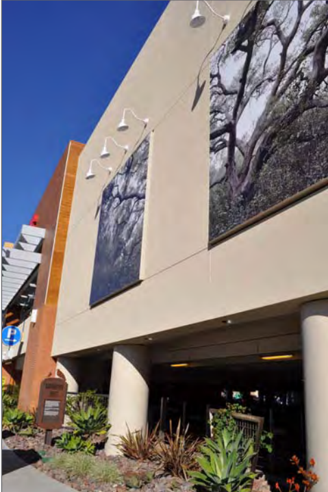
Walls may be made more visually interesting by incorporating art work or other surface articulation.
