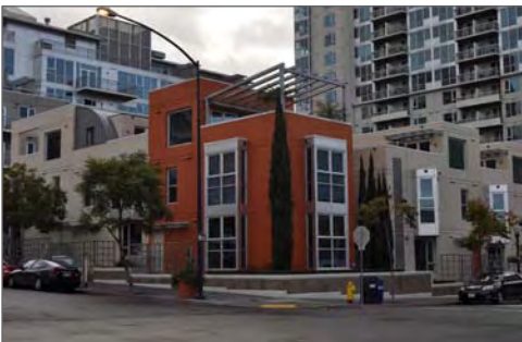
High quality materials are encouraged for residential buildings. Windows should allow for a shadow line and depth.
