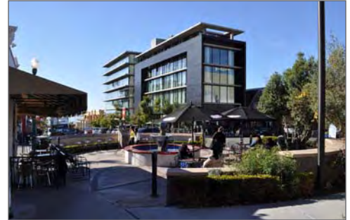
Open space with pedestrian amenities such as seating, shade, landscaping, and water features are ideally located at intersections.
