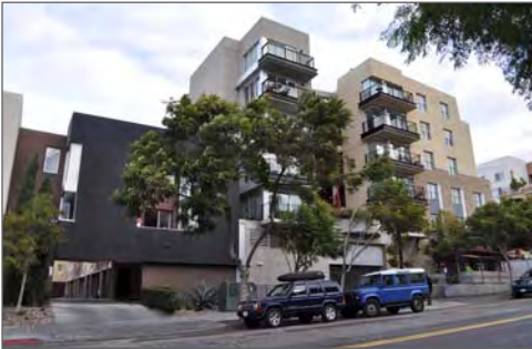
Garage openings should adhere to the overall aesthetic of the building's architecture.
