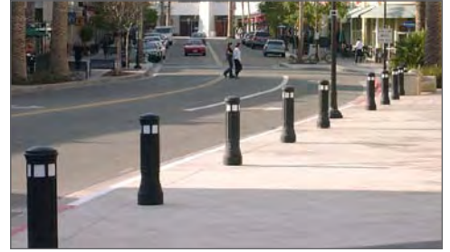
Lighted bollards provide pedestrian-scale lighting by illuminating a safe path of travel.
