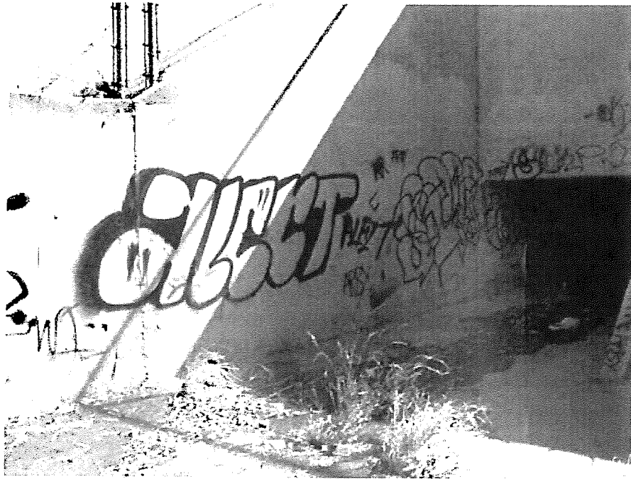
GRAFFITI IN CHANNEL - BEFORE
