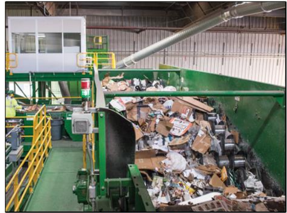
PHOTO 6: Material Recovery Facility (MRF)
