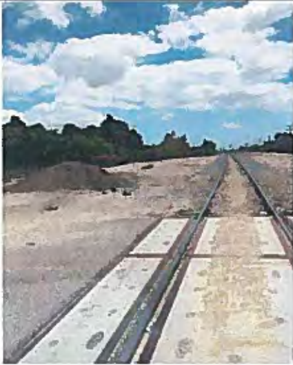
Illegal dumping – Train Tracks Adjacent to Athens Park
