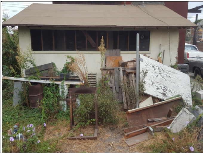
21. North side of empty structure.
