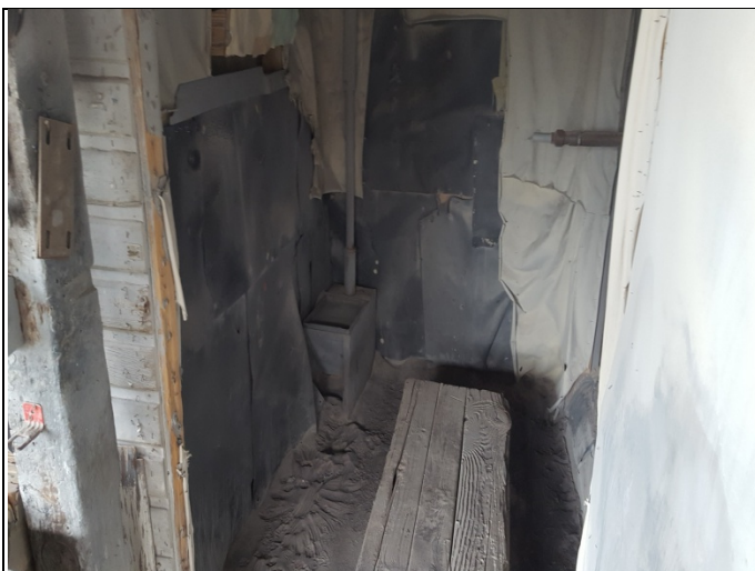
17. Former sand blasting area.
