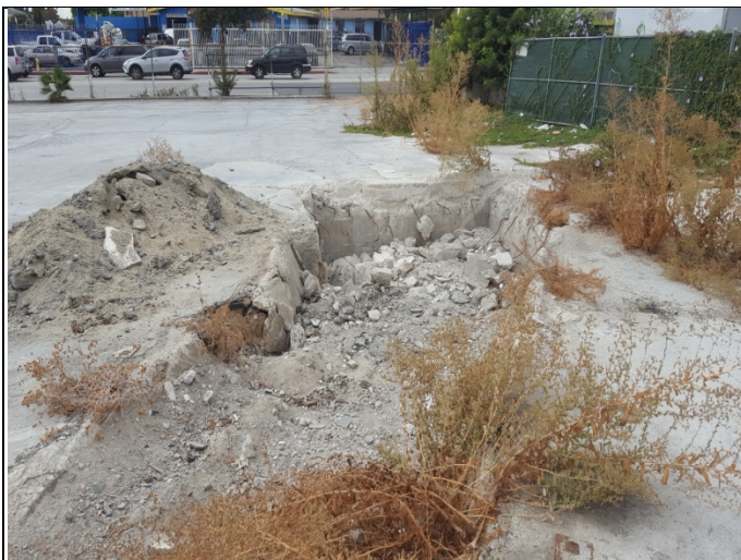
9. Excavation on the subject property in area of former structures.
