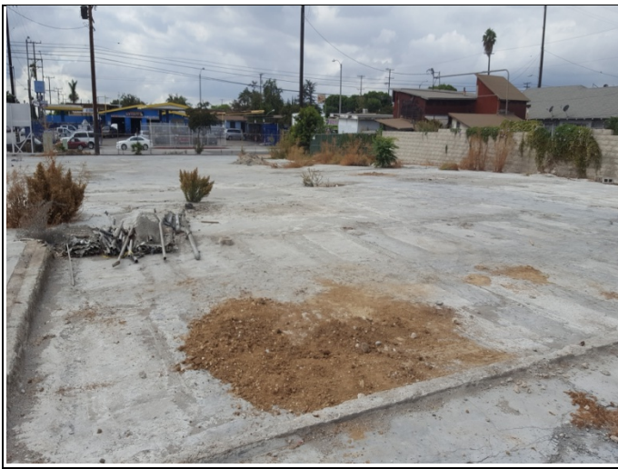
7. Looking south across the east side of the property in the location of the former structures.
