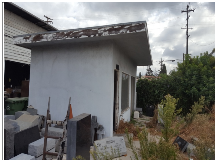
10. Office structure on the southwest side of the property.
