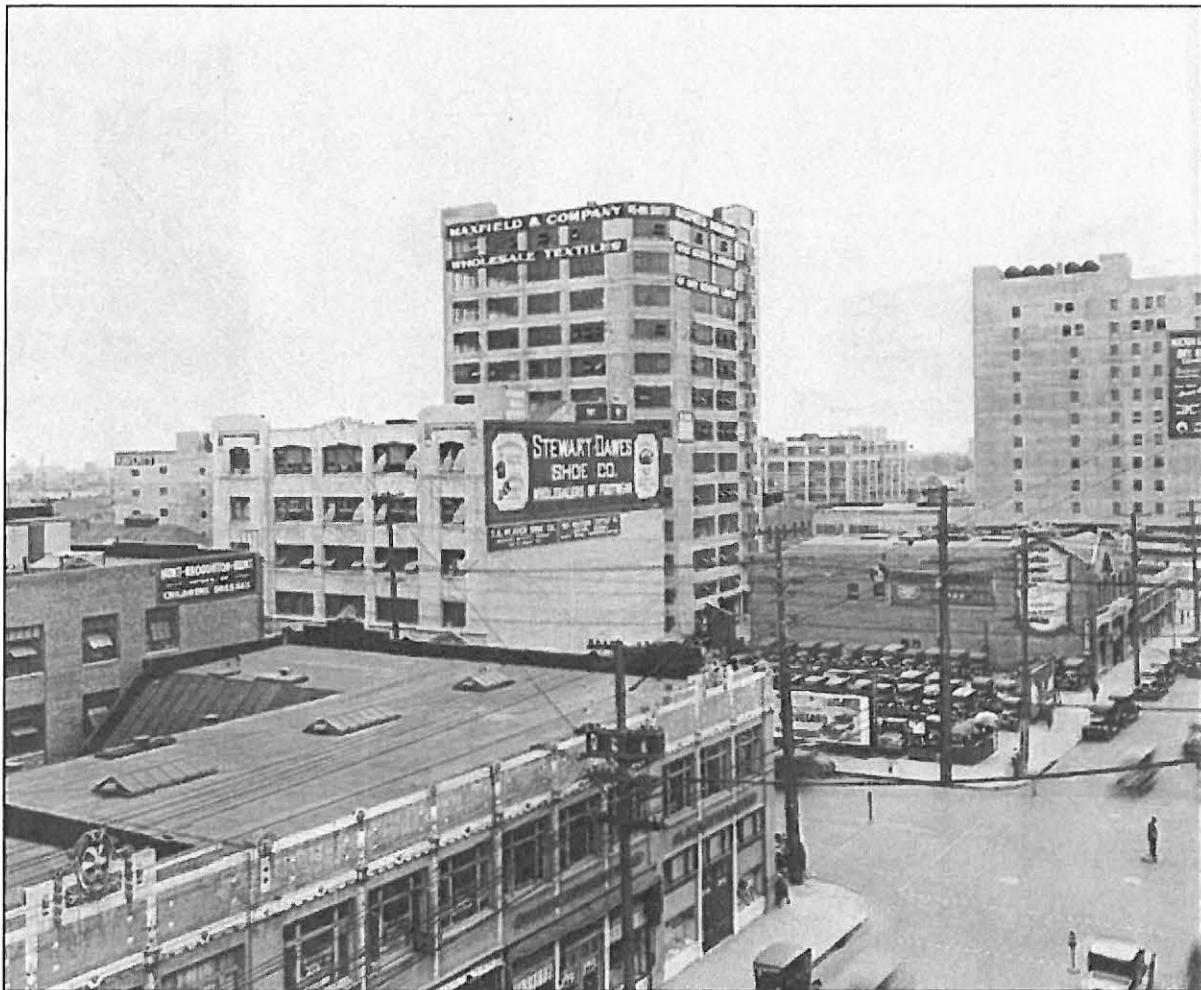
Figure 3. Maxfield Building, view of north and west elevations shortly after construction, note painted signage reading “MAXFIELD & COMPANY WHOLESALE TEXTILES” (USC Libraries Special Collections circa 1925)
