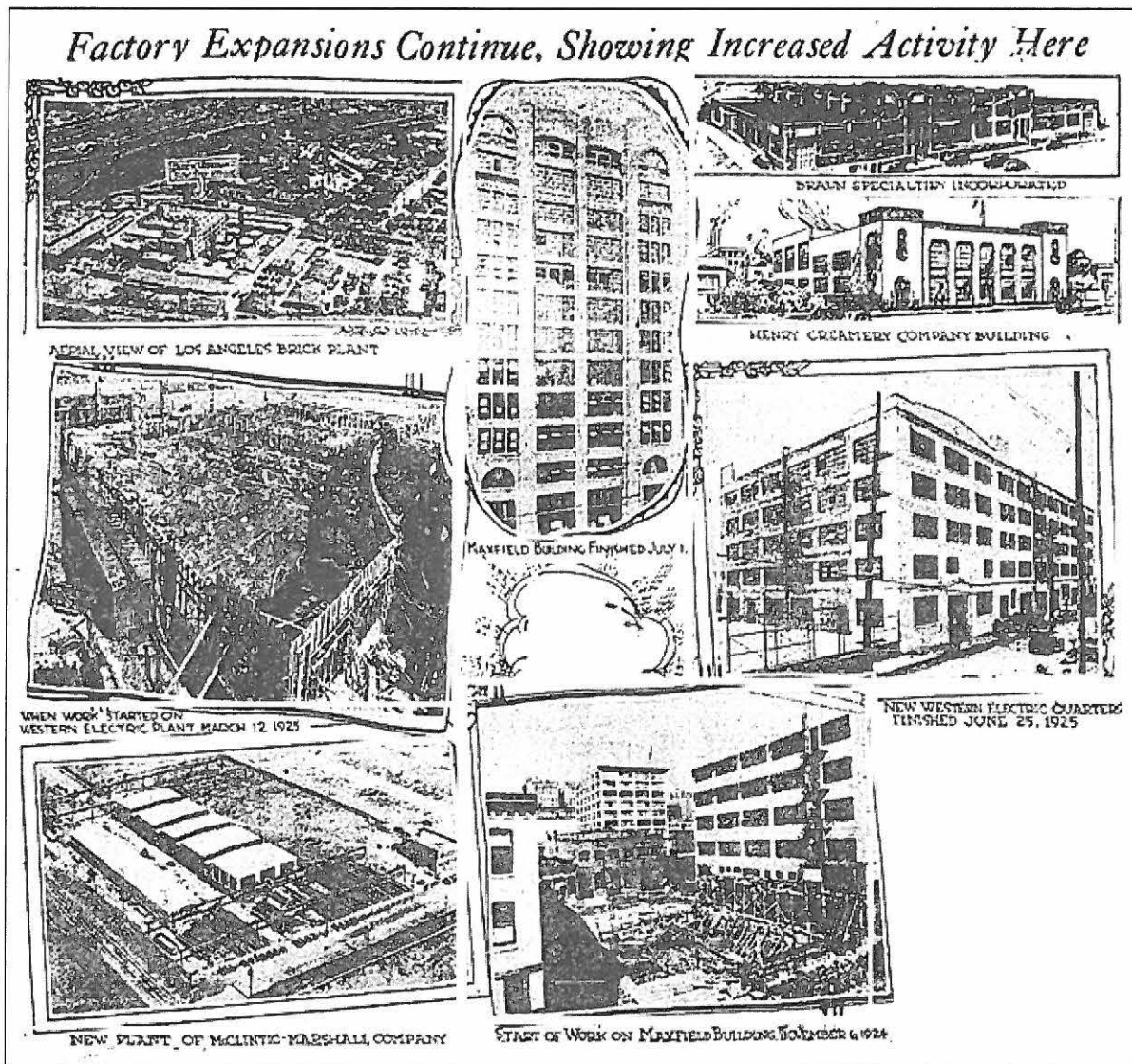
Figure 2. Article on factory construction in Los Angeles with photos of Maxfield Building construction (lower right) and completion (center top) ( Los Angeles Times , 1925)
