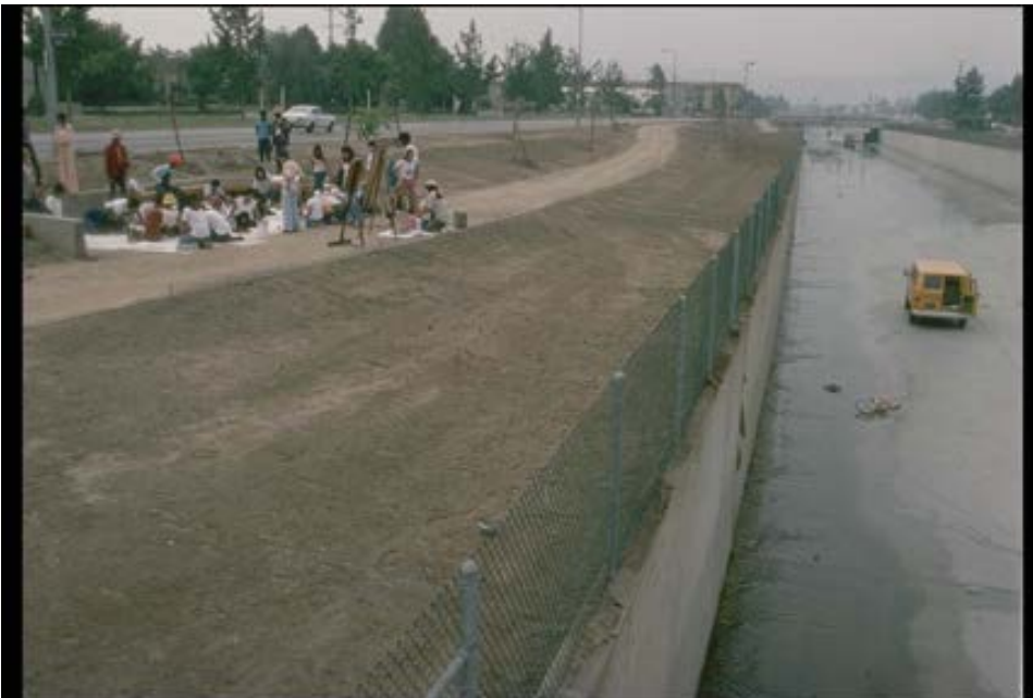
Figure 2 Meeting next to the Tujunga Flood Control panel, prior to painting, c. 1976 (Courtesy SPARC)
