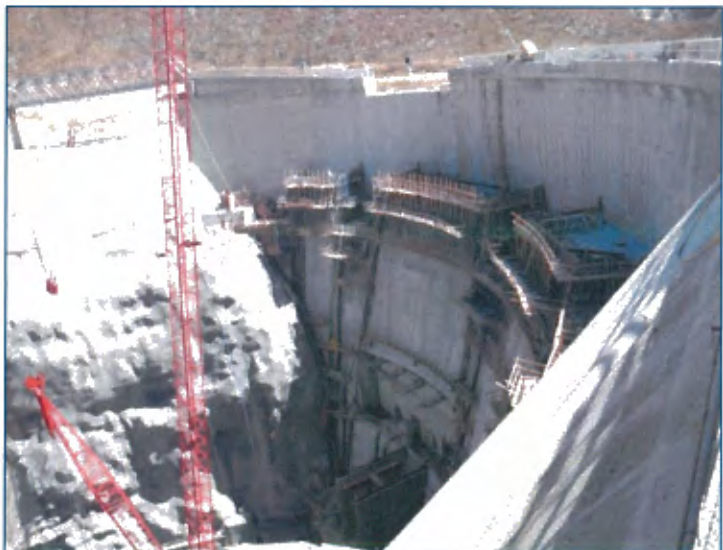
Construction of Big Tujunga Dam Seismic Rehabilitation - 2008
