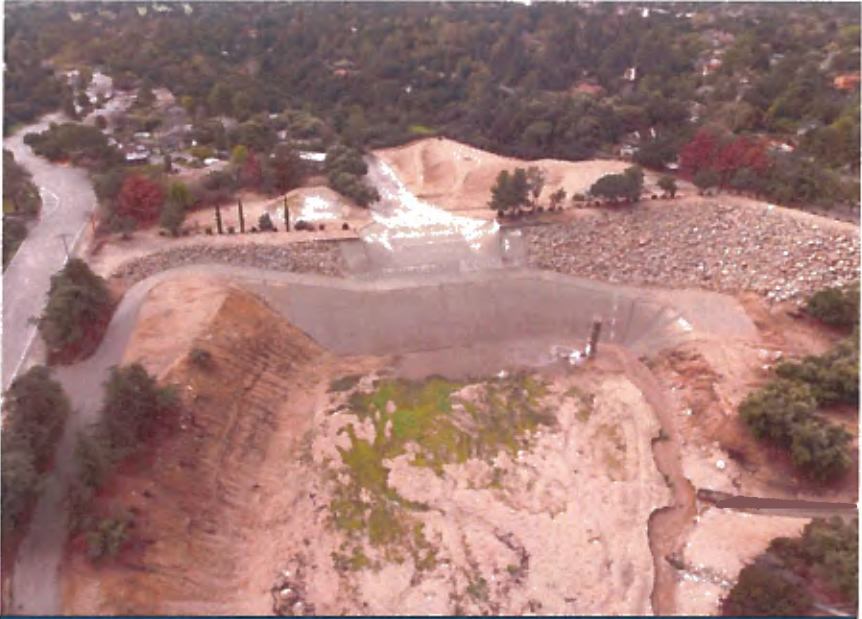
Rubio Debris Dam
