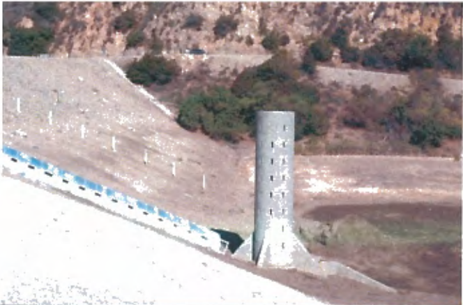
Little Dalton Debris Dam - Upgraded Outlet Tower 2013
