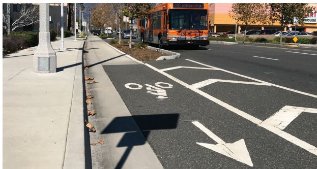
Separated Bikeways provide physical separation between bicyclists and traveling motorists.
