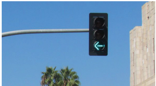
Left Turn Signal Phasing provides a green arrow for left turning vehicles while stopping conflicting vehicles and pedestrians.
