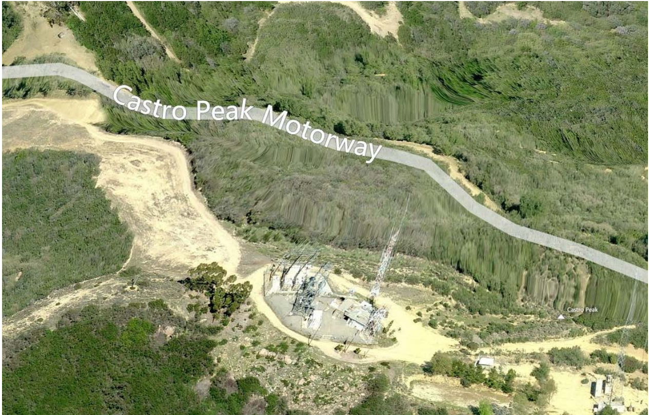
County of Los Angeles Castro Peak Telecommunications Site Castro Peak Motorway Malibu, CA 90265
