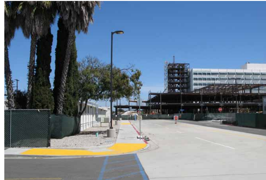
New Emergency Department construction
