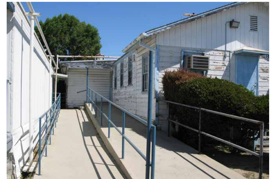
Accessible ramps interfacing with WWII modular buildings
