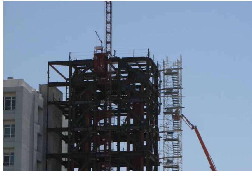
New elevator connection to Existing Hospital Tower
