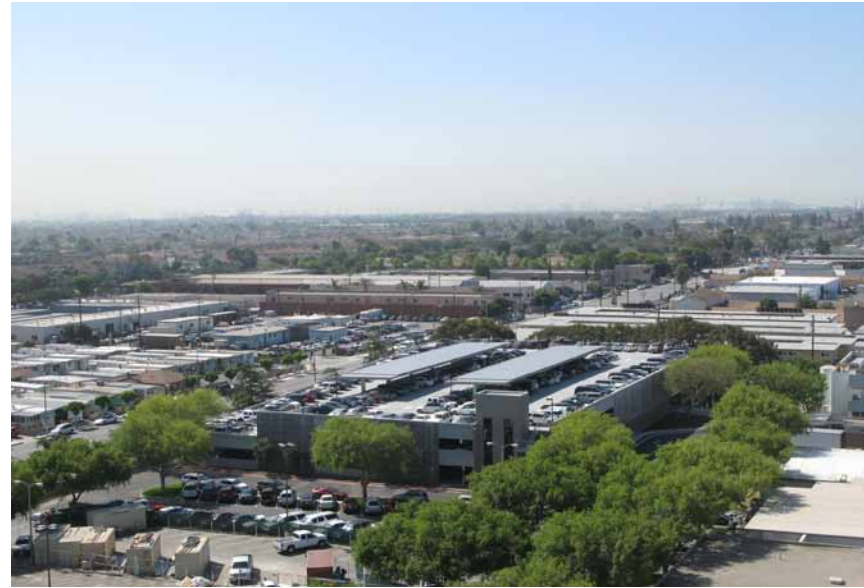
Existing parking structure with Photovoltaic cells
