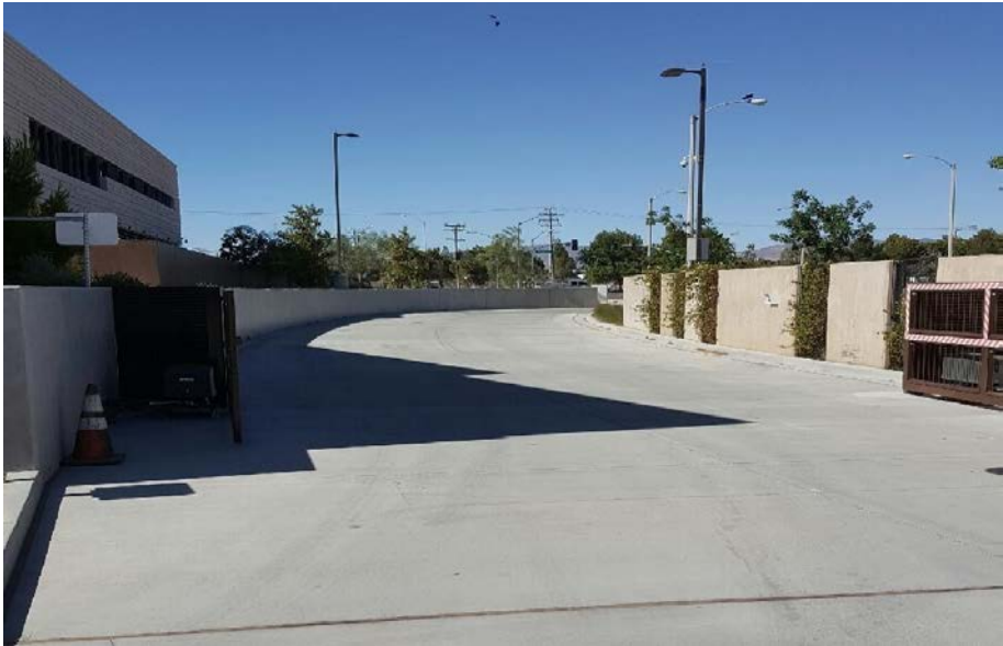
3 rd Street Entrance
