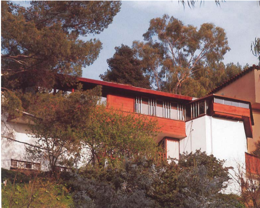
View of west façade, facing southeast (Photo credit: Alan Weintraub, The Architecture of John Lautner by Alan Hess, date of photograph unknown)
