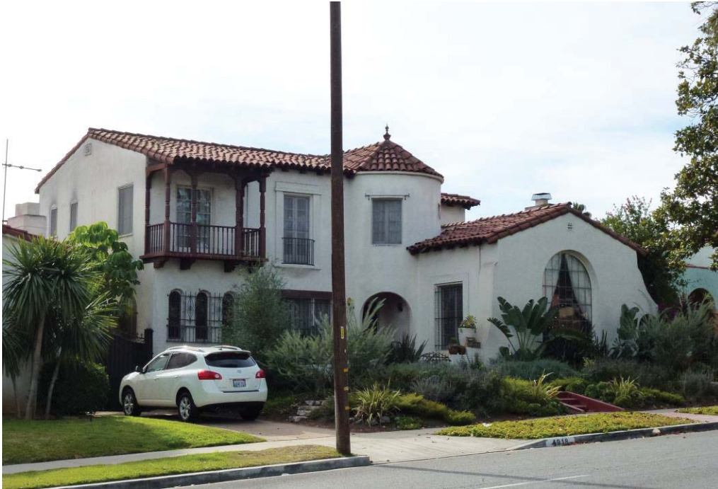
Figure 8. View toward the southwest of the north and east facades. Source: ASM Affiliates: Date: December 3, 2015.
