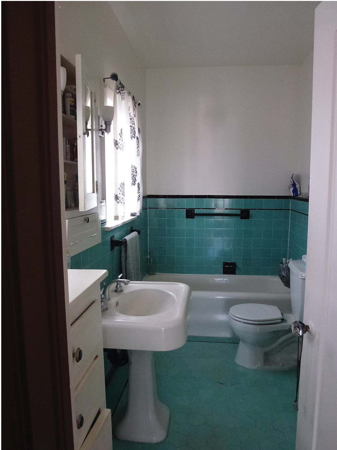
Figure 19b. Interior view of additional second-floor bathroom. Source: ASM Affiliates; Date: December 3, 2015.
