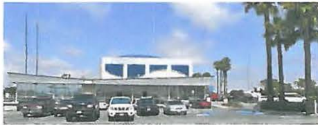
WEST ELEVATION FACING PARKING LOT BEFORE
