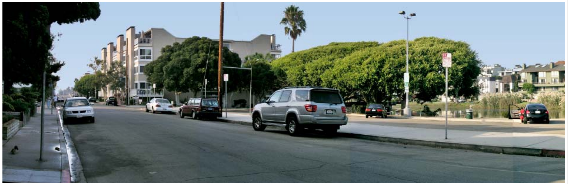
City of Los Angeles Venice Pumping Plant Dual Force Main Project
