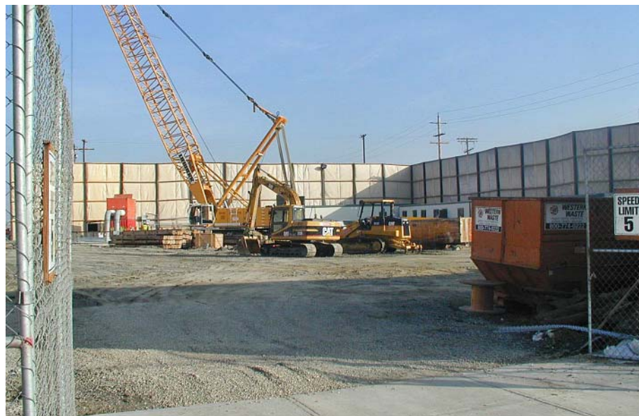
Clockwise from Top: Construction Equipment for Typical Cut-and-Cover Construction. Sound Barriers, Seen from Street and from within Shaft Construction Area. Shaft, within Sound Barrier.
