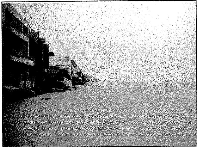
Figure 3. Beach Alignment (view to the south, north of the Channel).
