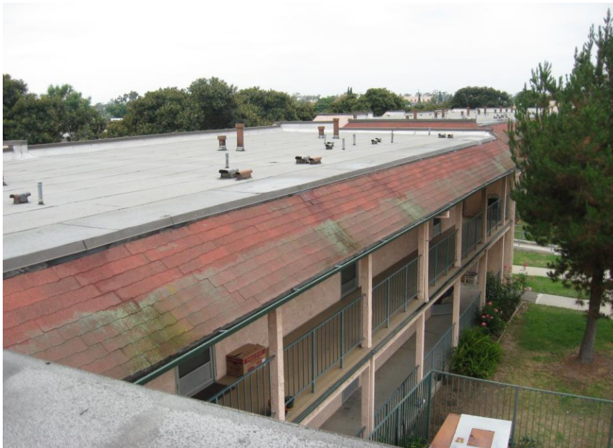
(2) Existing roof view of one of the four buildings.
