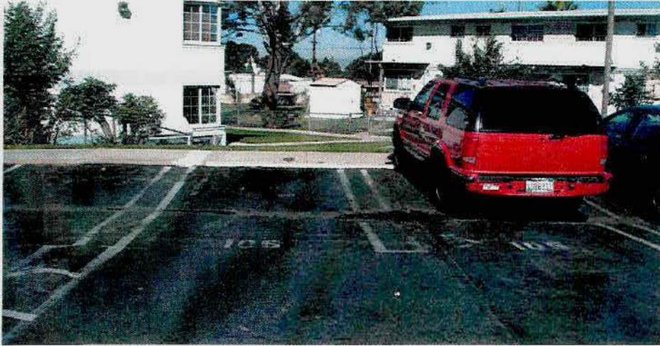
Ponding and excess oil
