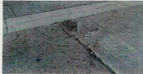
Concrete cracking
