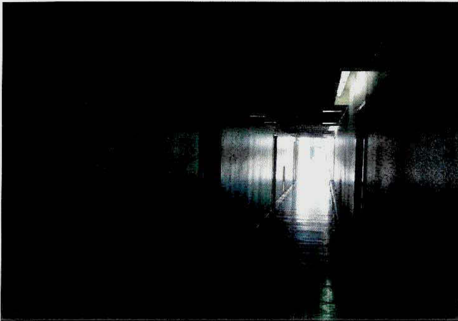
Internal breezeways - replacing & improving lighting. Painting walls and ceiling.
