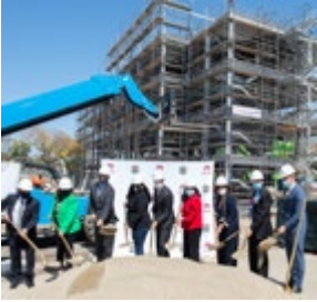
LAC+USC Medical Center Restorative Care Village groundbreaking
