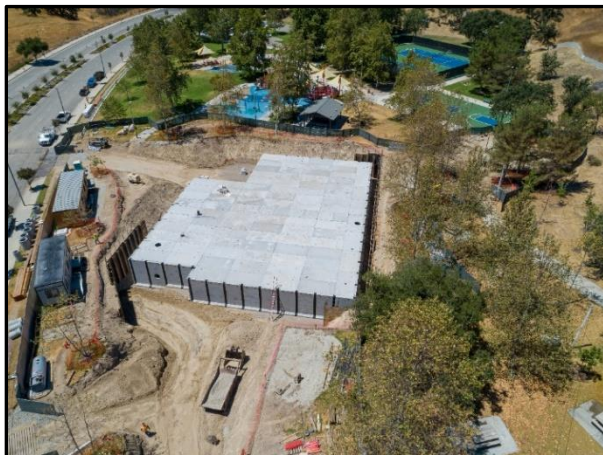
During construction, the grass was removed and a 145-ft by 108-ft cistern was built 25-ft below the ground.
