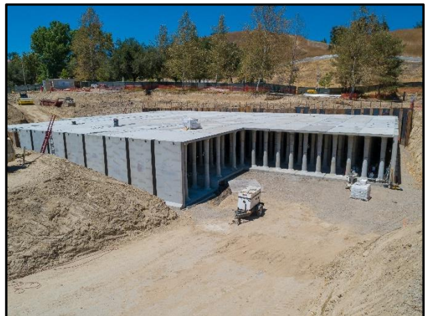
During construction, the grass was removed and a 145-ft by 108-ft cistern was built 25-ft below the ground.
