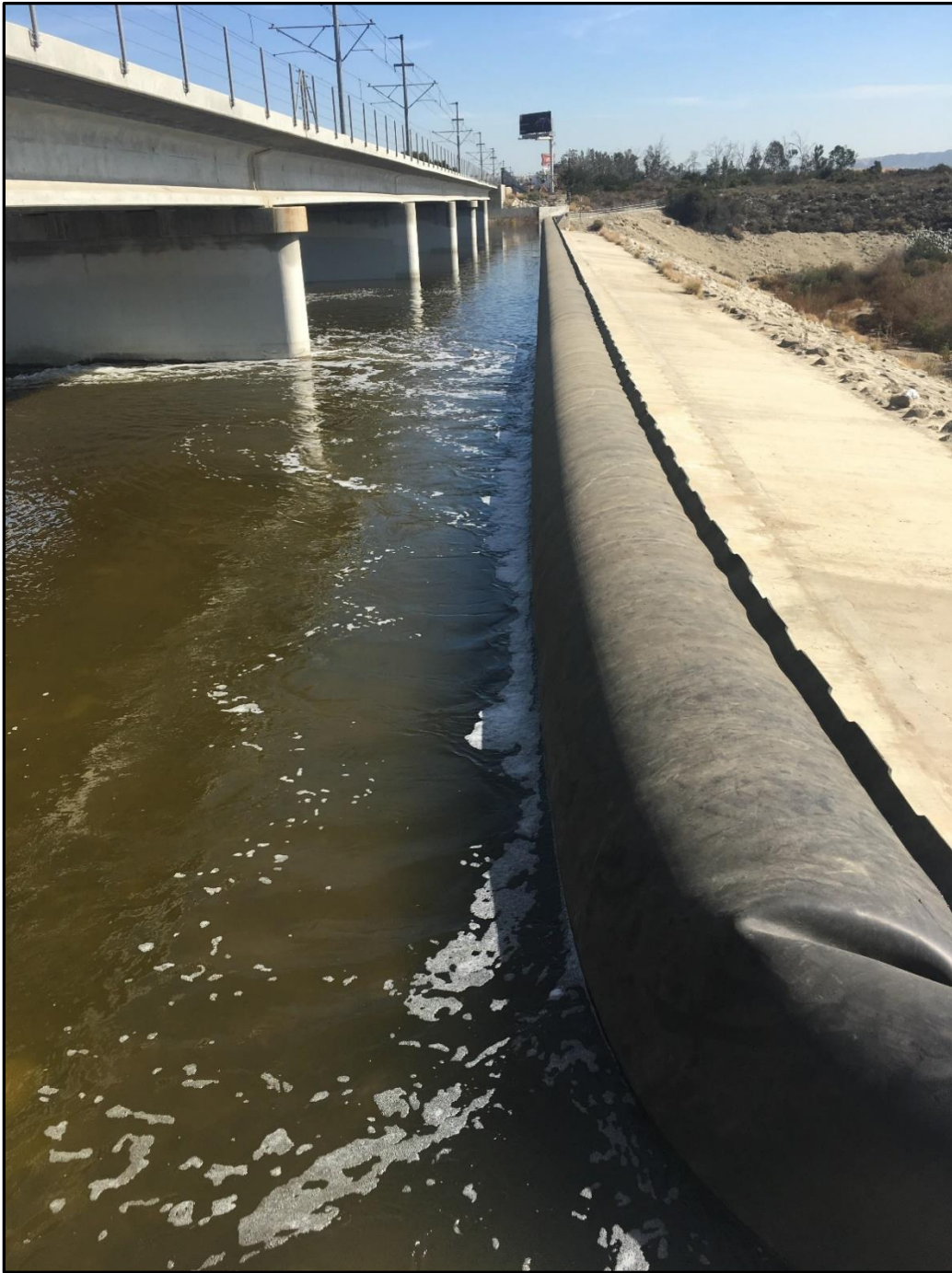
The new rubber dam was installed and inflated with water.
