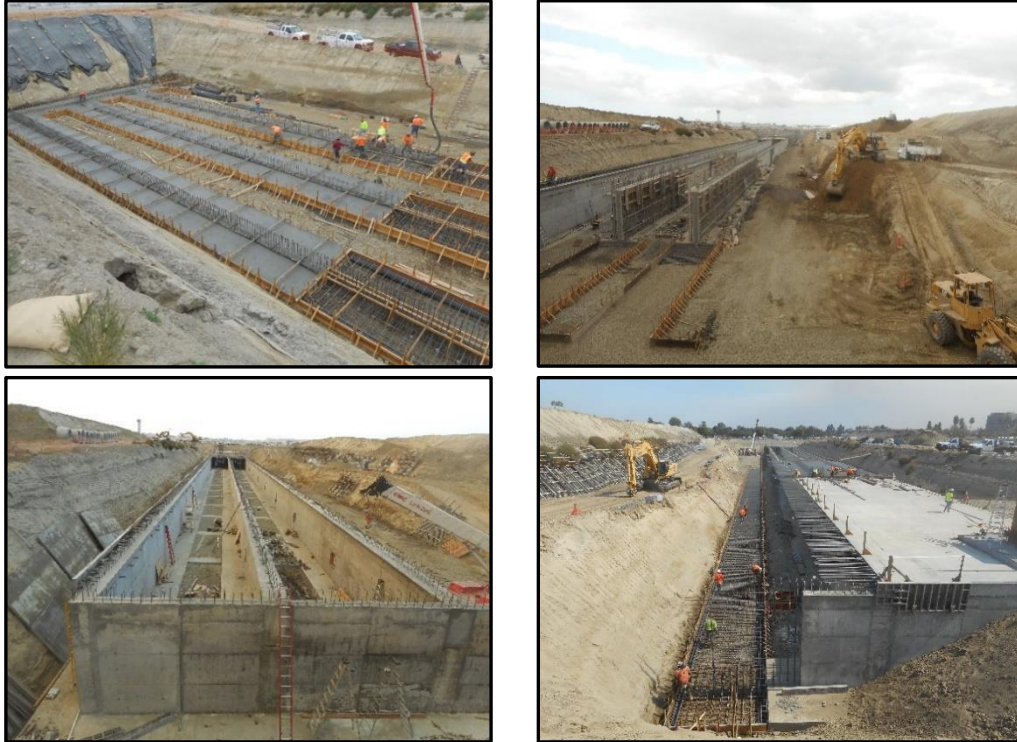
Infiltration gallery during construction
