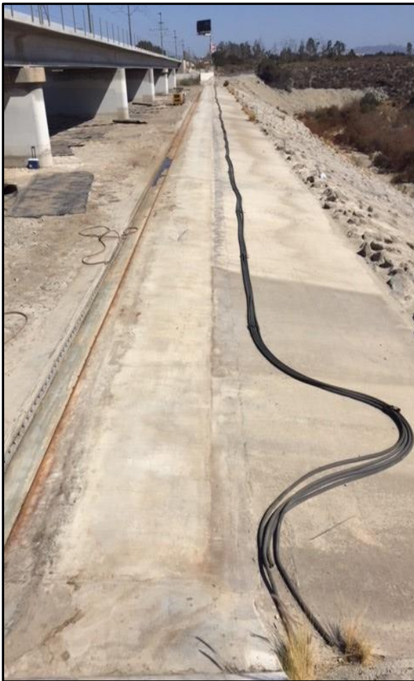
The old rubber dam was removed, and the new rubber dam was partially installed.
