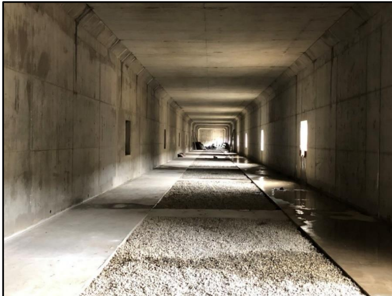
Infiltration gallery completed
