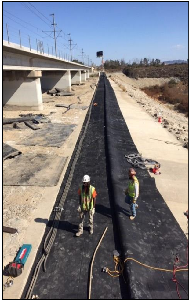
The old rubber dam was removed, and the new rubber dam was partially installed.
