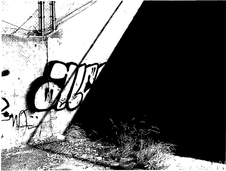
GRAFFITI IN CHANNEL - BEFORE
