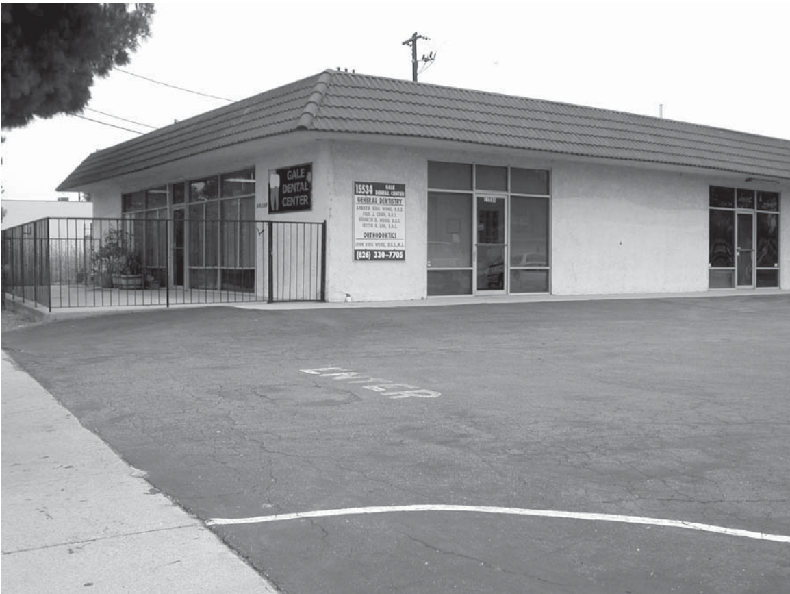
PHOTO 2. Building adjacent to project site on the west, facing east (June 5, 2003).
