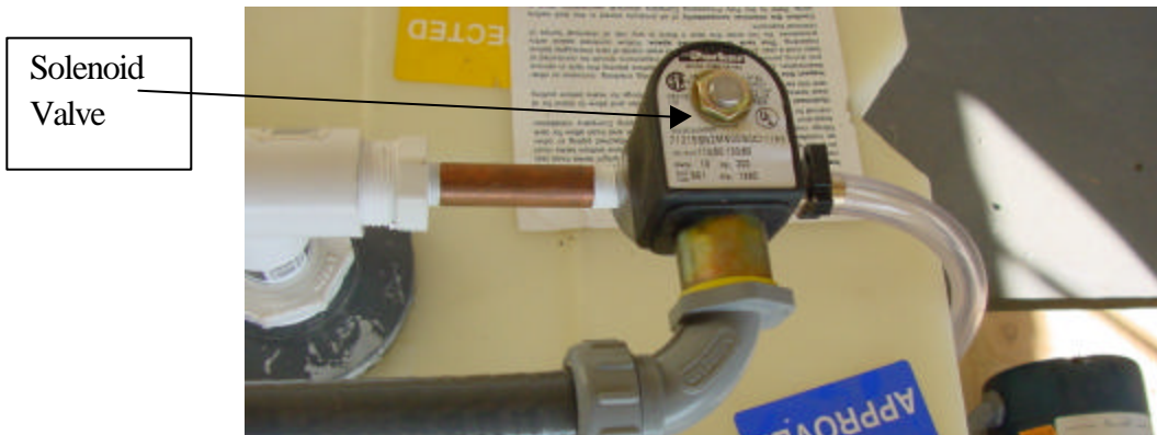
Figure 3: Normally closed solenoid valve
