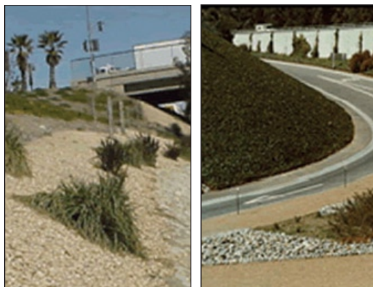
Public roadway projects - Gravel mulch involves the placement of loose evenly graded crushed or quarried rock on top of a geosynthetic fabric. The fabric prevents plants from rooting and the weight and porosity of the gravel keep the fabric in place and allow for percolation of water and air. http://www.dot.ca.gov/hq/LandArch/roadside-detail-gm.htm
